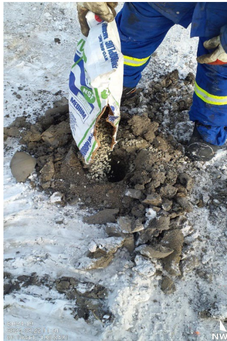
Photo 25 – Backfilling BH24-19 with bentonite (22 March 2024).
