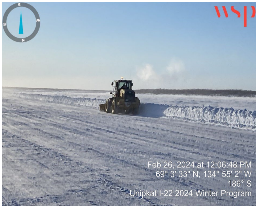
Photo 13 – Ice Road Construction - Loader widening road between KM-80 and KM-85 (26 February 2024).
