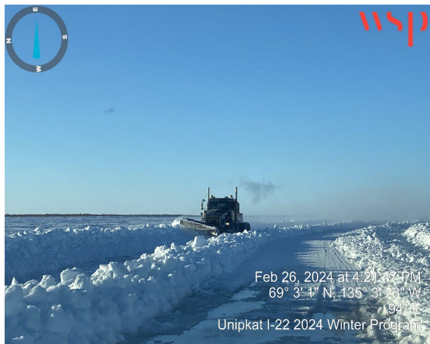
Photo 14 – Ice Road Construction - Tandem axle plow truck opening section of road between KM-85 and KM-92 (26 February 2024).
