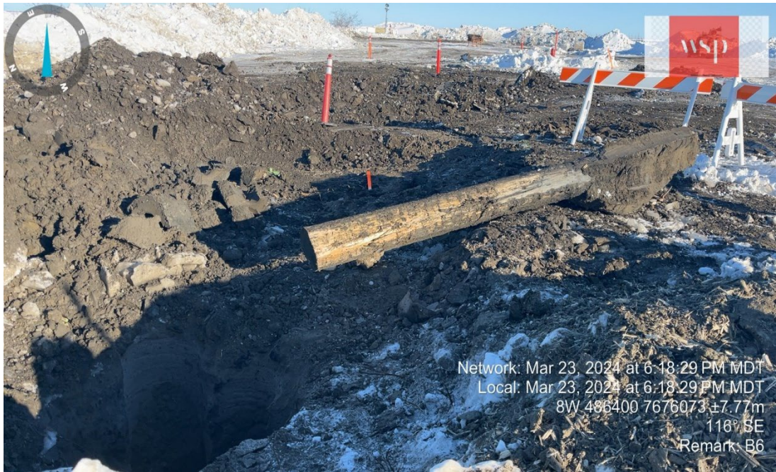
Photo 23 – Wood Piling Removal – Extracted intact wood pile (23 March 2024).
