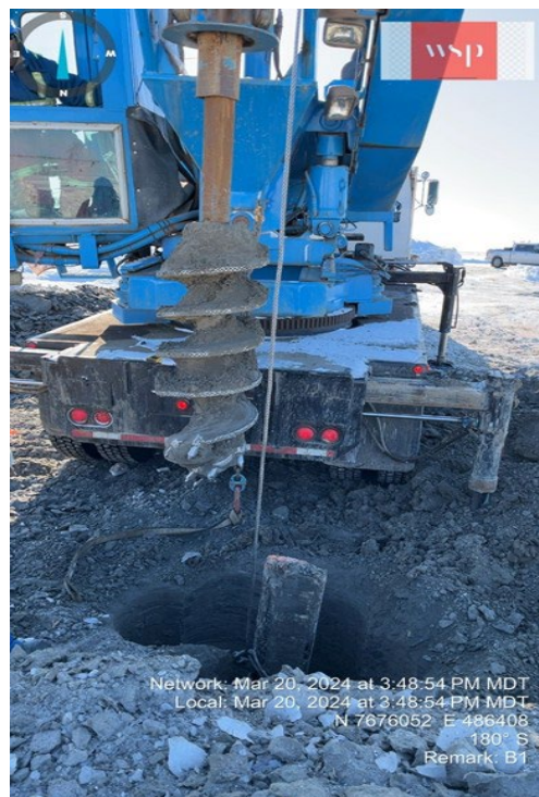
Photo 22 – Wood pile removal using Texoma Auger drill rig V-017 at northeast of the Site (20 March 2024).
