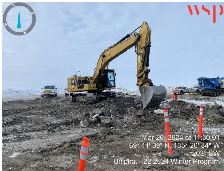
Photo 24 – Wood Piling Removal - CAT 330 exposing existing pilings (26 March 2024).
