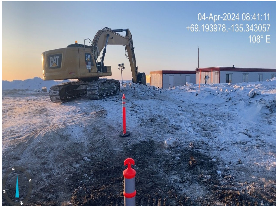
Photo 29 – Leveling the surface around BH24-01 and -02 to create safe drilling rig access (4 April 2024).
