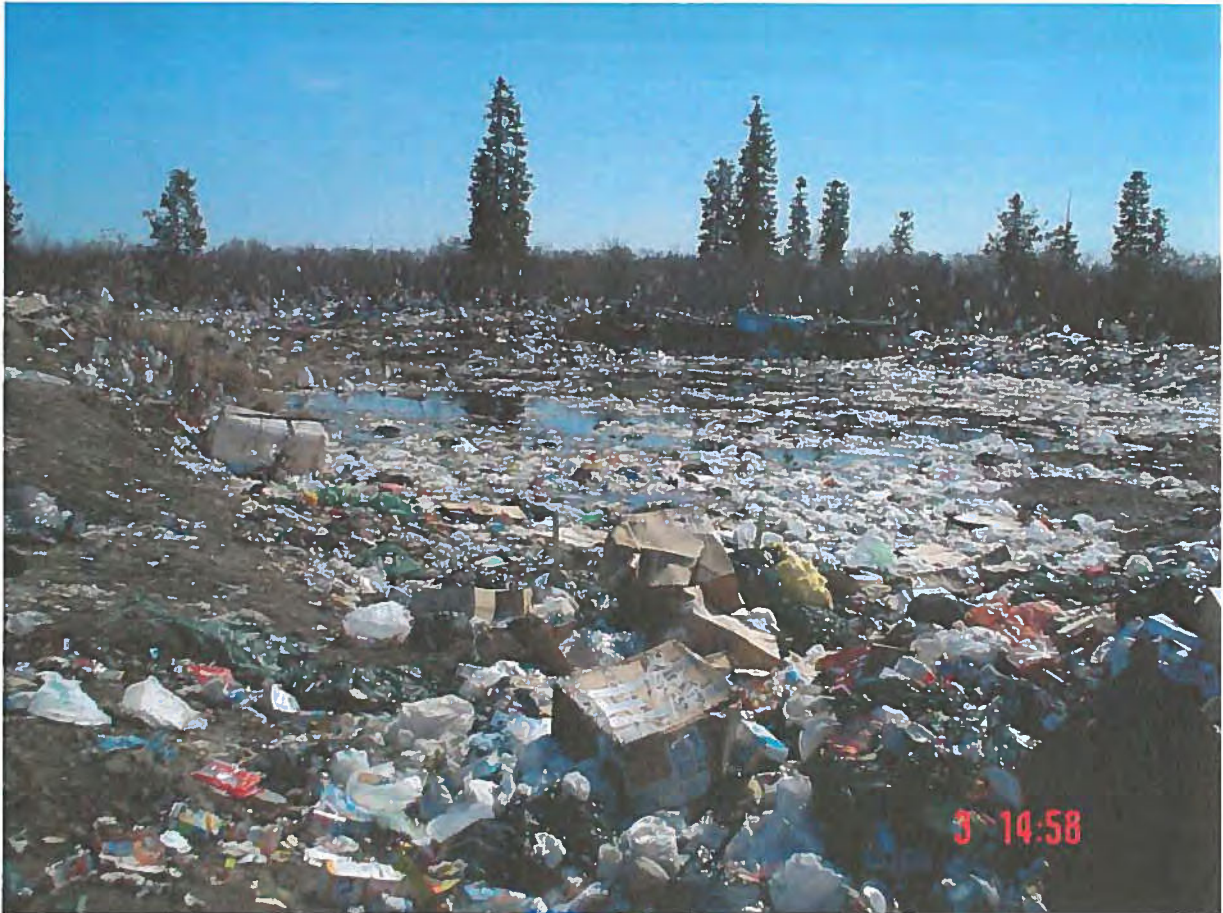
Photo 8: Standing Water in Landfill #2
