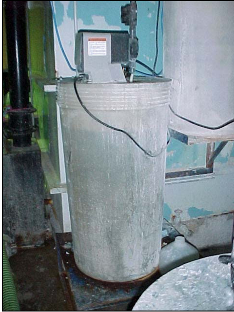
Photo 51 Polymer injection system for Waterboy.
