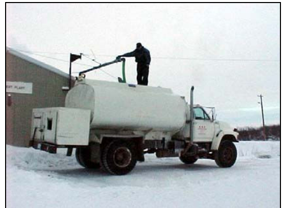
Water Treatment Plant & truckfill operation
