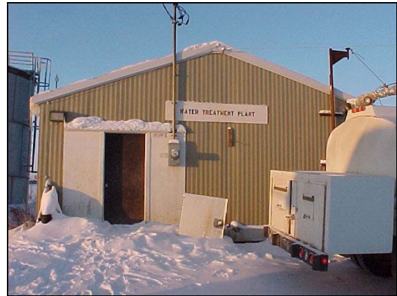
Photo 7 Water Treatment Plant.
