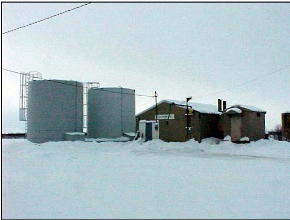
Photo 6 Water Treatment Plant.
