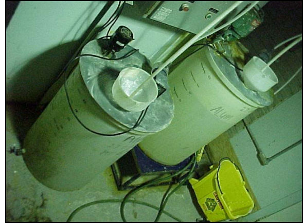
Photo 52 Powdered alum injection systems (FTC & Waterboy).
