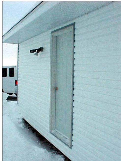
Photo 76 Side entrance with security light.
