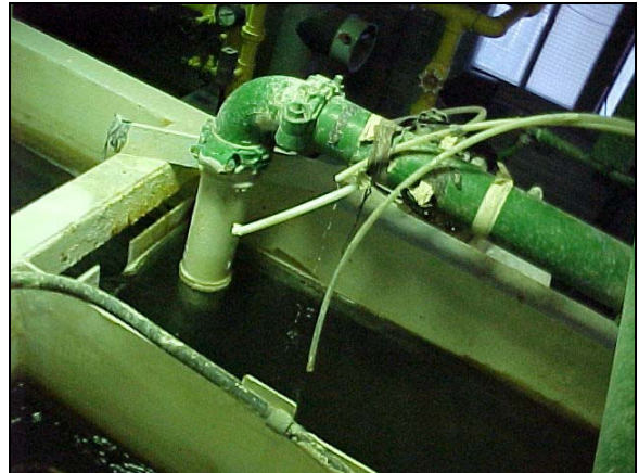
Photo 40 Flash mix chamber @ Waterboy with polymer and alum injection.
