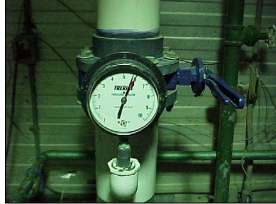
Photo 5 Level gauge for storage tanks.
