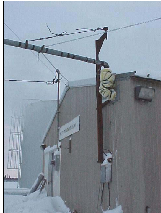
Photo 89 Truckfill arm – modification under way.
