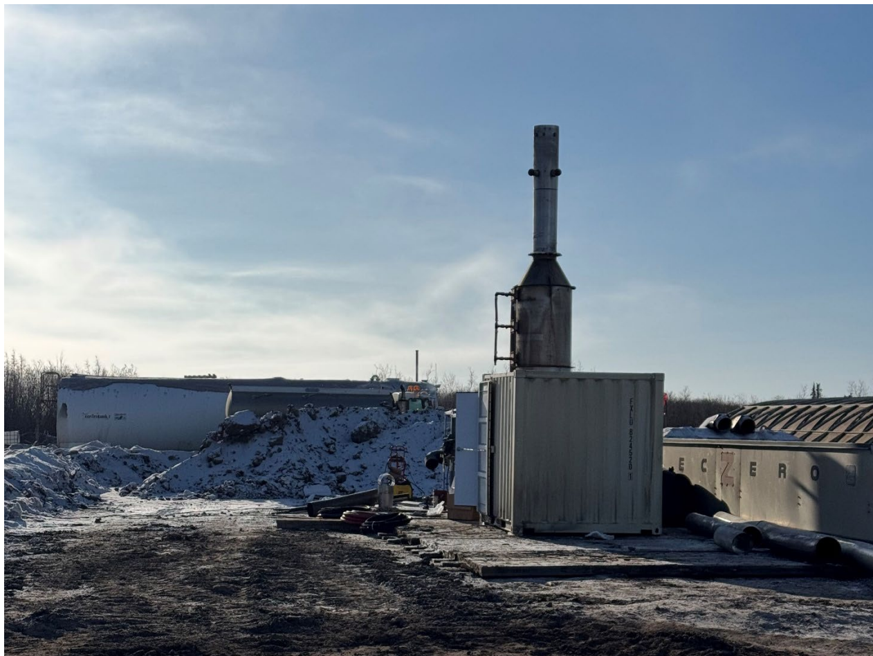
Photo 1: A quench tower set up during Northern Canada Winter Operations
