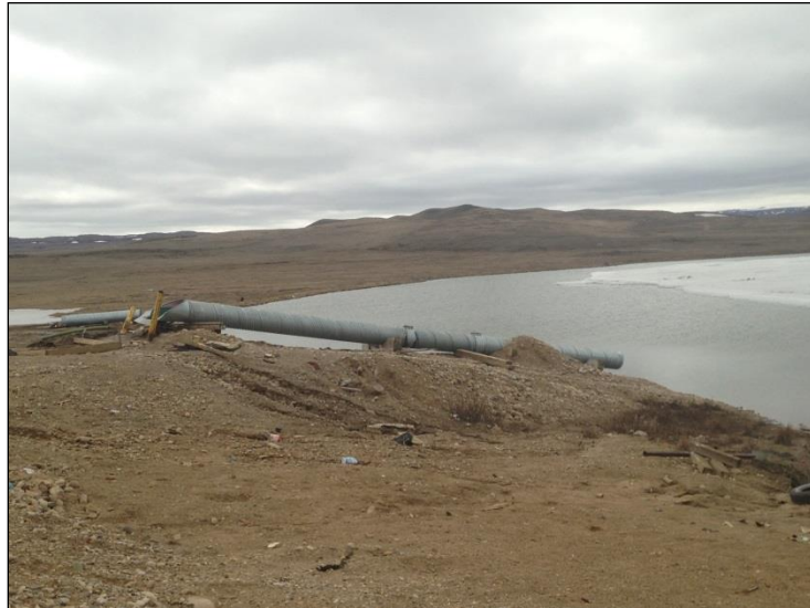
Figure 2: Paulatuk Discharge Chute (2015)
