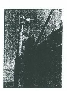
Photo 28. A camlock hose is attached to the top of the piping (indicated by white arrow) in order to fill water truck.
