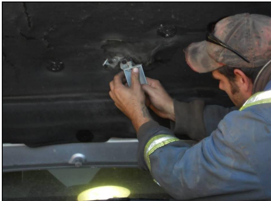
Figure 3.17: Example of Removing Light Assembly Containing a Mercury Switch
