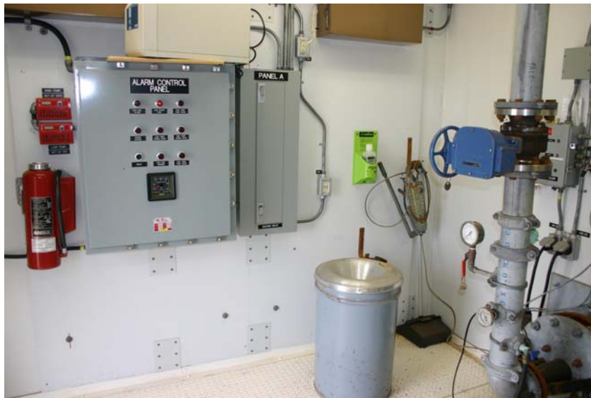
Inside Pump House
