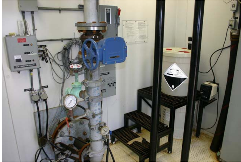
Inside Pump House
