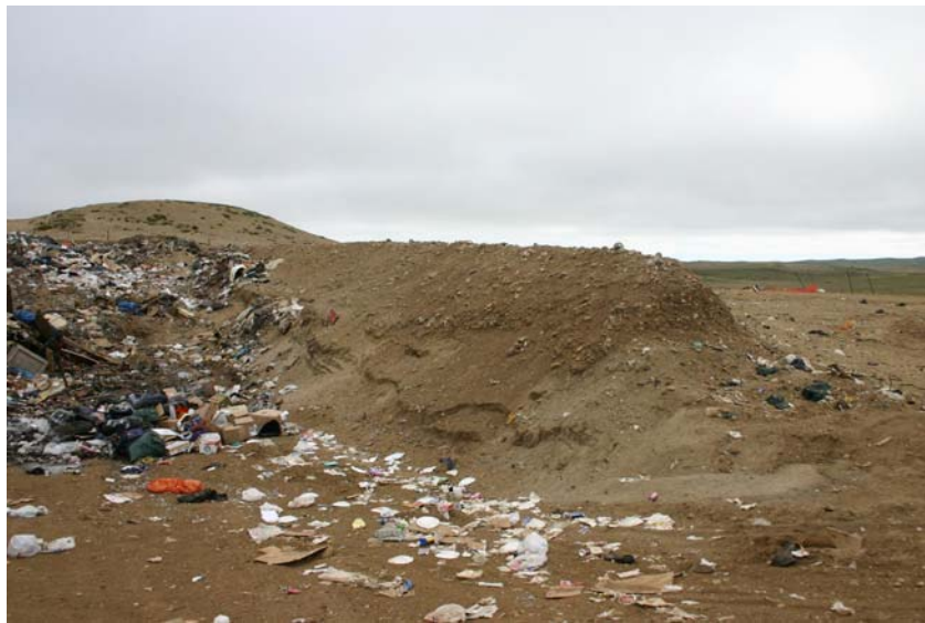
Waste disposal cell currently being filled
