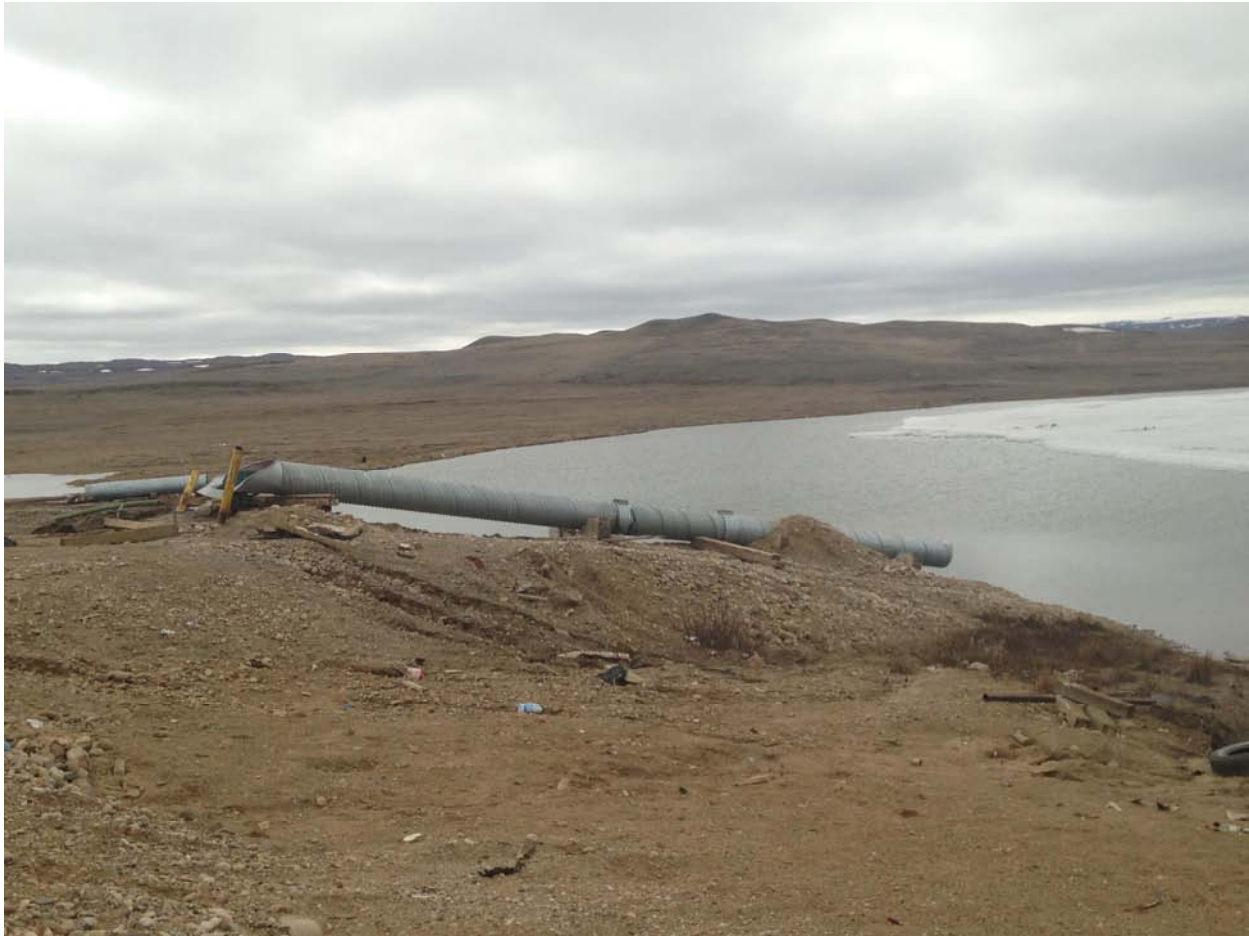
Figure 2.1 Paulatuk Discharge Chute
