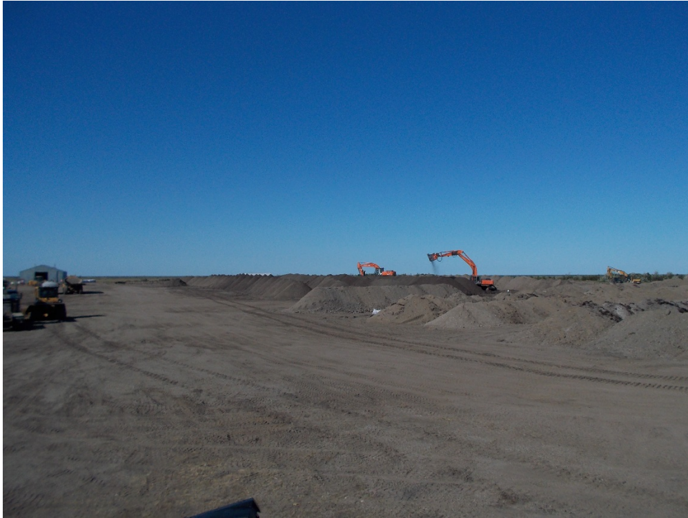
Photograph 3: Impacted soil windrowed and being treated with an Allu bucket (August 6, 2016).
