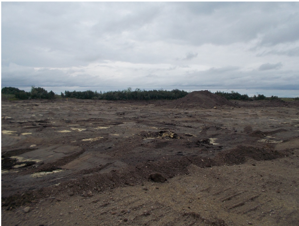
Photograph 2: View northwest of Zone 2 excavation (August 29, 2016).
