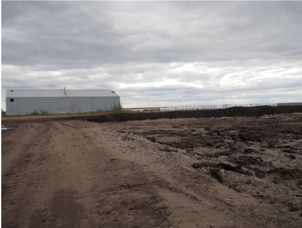
Photograph 5: View south of shed #1 building in good condition and soil bags prepared for removal off-site (August 19, 2016).
