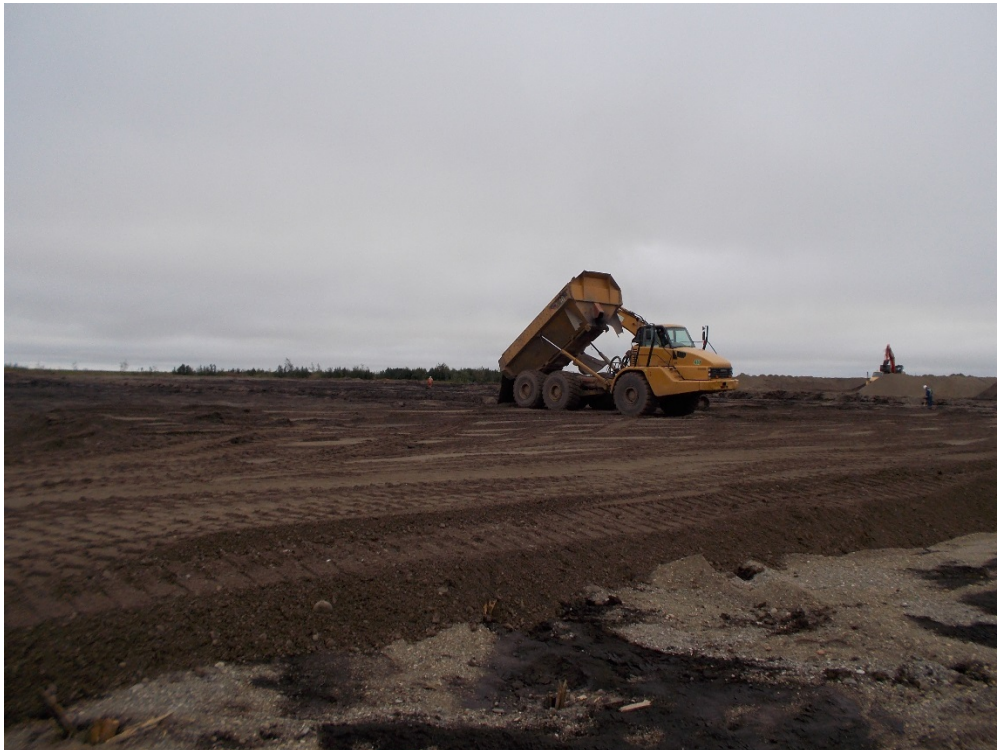
Photograph 4: View northeast of excavated area being backfilled with treated soil (August 5, 2016).
