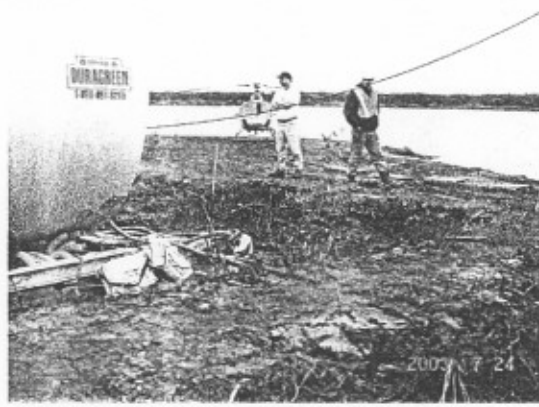
Figure 2. Southeast corner of containment berm.
