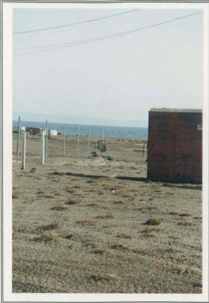
Photo # 5: Power Line and Pipe Line used to transport electricity and fuel from the beach area to the garage and tank farm. Red steel shack on right contains 1-400 gal. tank.
