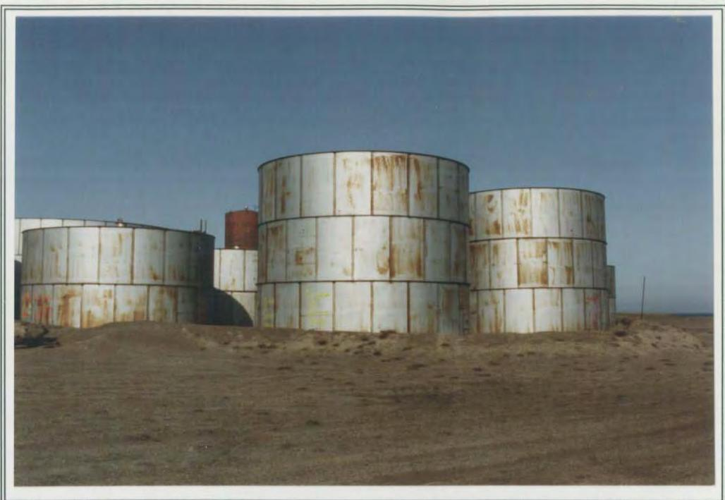
Photo # 19 Area # 4. Bolted tanks, 2 and 3 tiered. Note red tank.
