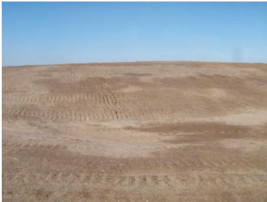
Photograph 21 – Straight-side of Disposal Area 1 by Landfill C. Erosion channels visible (Section 3.1.11).
