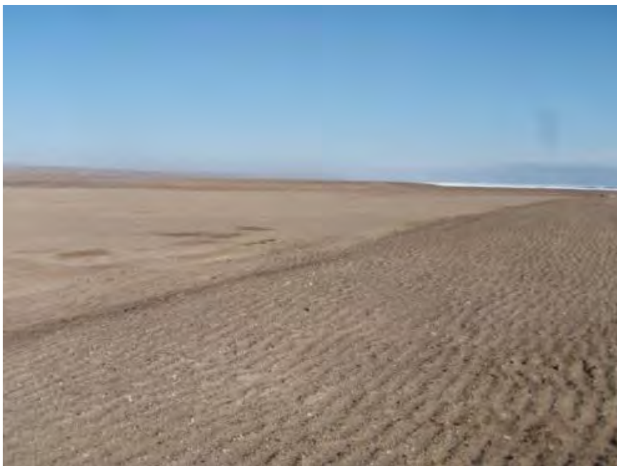
Photograph 14 – Northern, unarmored slope of Landfill A. Hydrocarbon staining is evident just off the landfill cap (Section 3.1.7).
