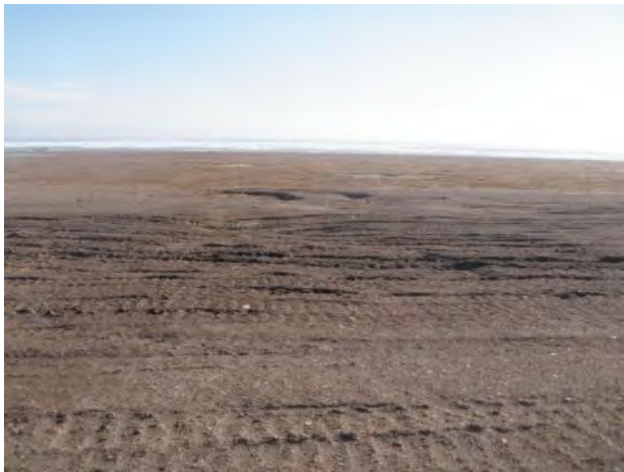
Photograph 24 – Area of settlement south of Disposal Area 2 (Section 3.1.11).
