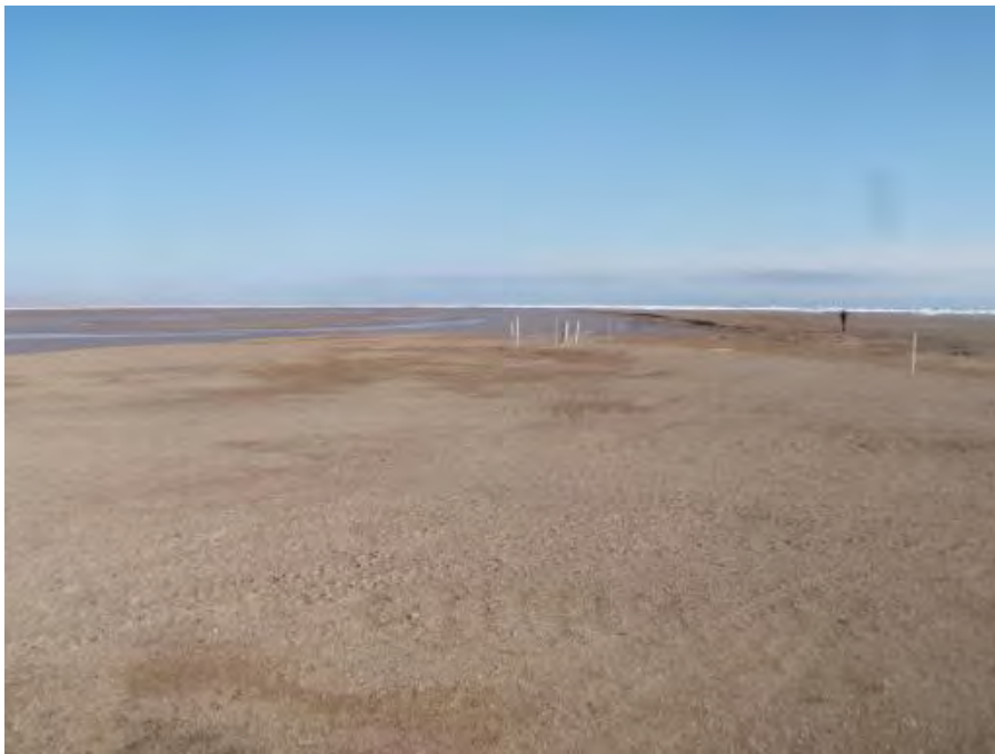
Photograph 7 – Apron Area. Thermistor T09-02, MW09-01, MW09-02, MW09-03, and MW09-04, looking north (Section 3.1.2.3).
