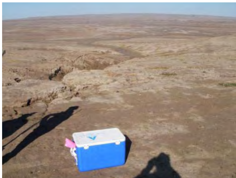
Photograph 22 – Drainage/Erosion channel west of Disposal Area 1. Mr. Arey indicated that erosion had occurred in this area (Section 3.1.11).
