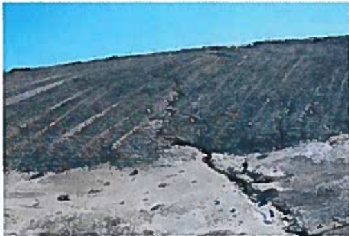
Figure 3 Water erosion running down slope towards area drainage which leads to Unnamed River.
