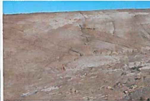
Figure 4 The borrow areas disturbance to permafrost without full restoration continues to have slumping and subsidence.
