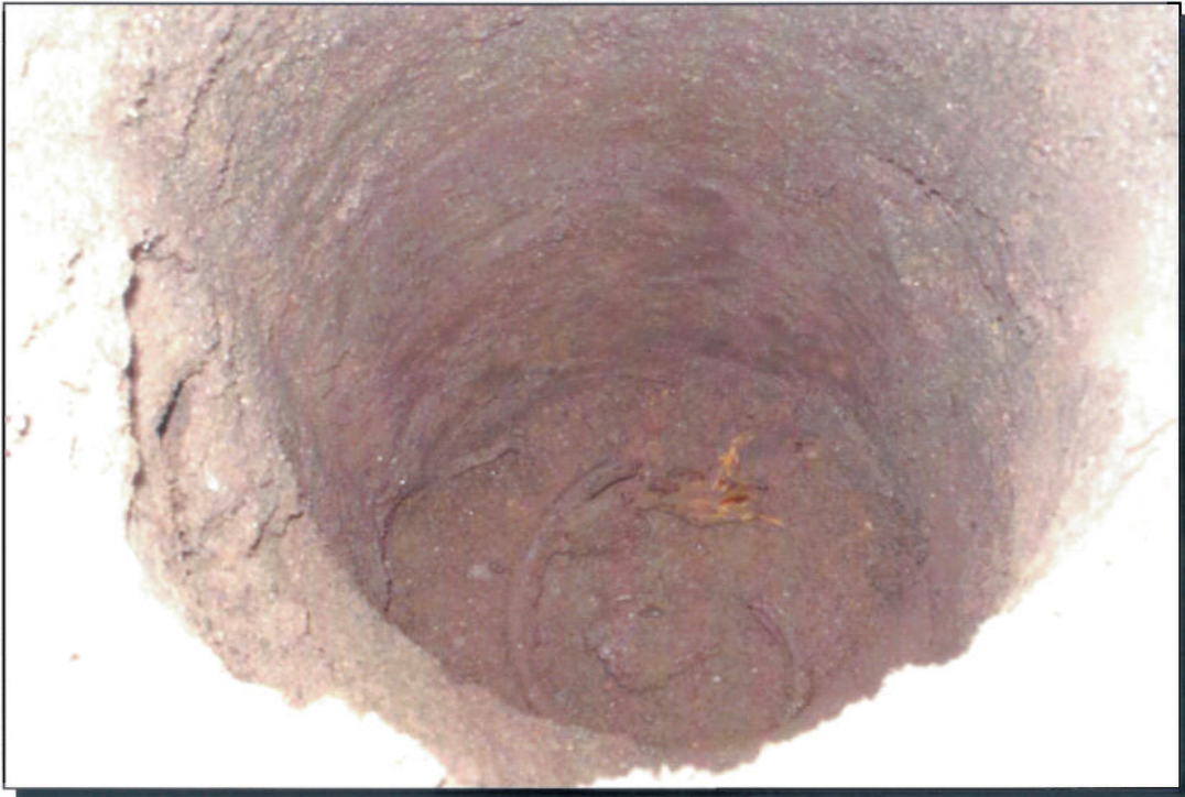
Photo 23 Existing Landfill C – wood and metal at the bottom of testpit
