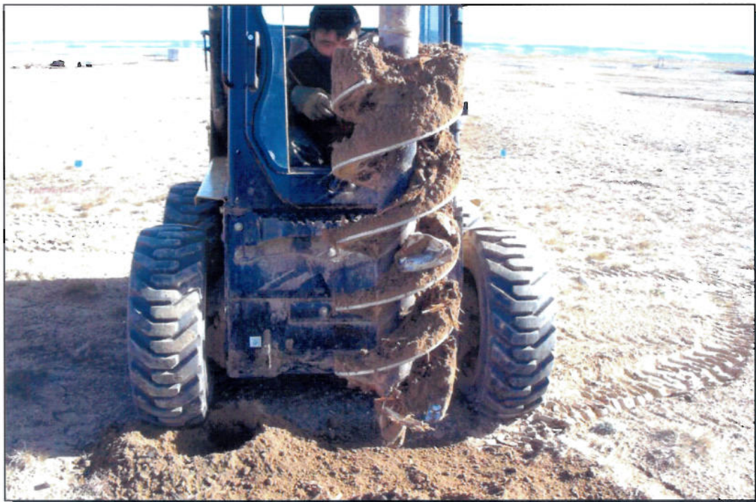
Photo 22 Existing Landfill B – wood and metal at about 0.3 m below grade
