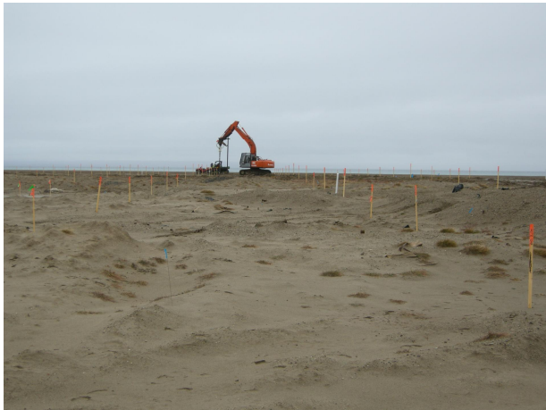
Photograph 39 ↑ Airstrip Landfill Area
