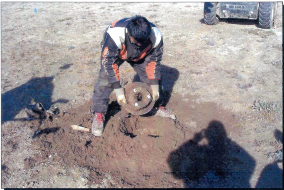
Photo 24 Existing Landfill C – debris encountered at about 1 m below grade
