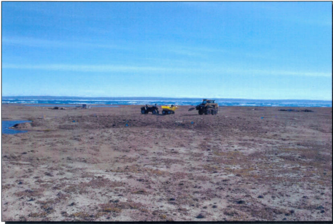
Photo 21 Existing Landfill B
