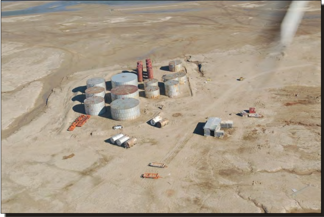
Photo 1 Aerial oblique of tank farm area.
