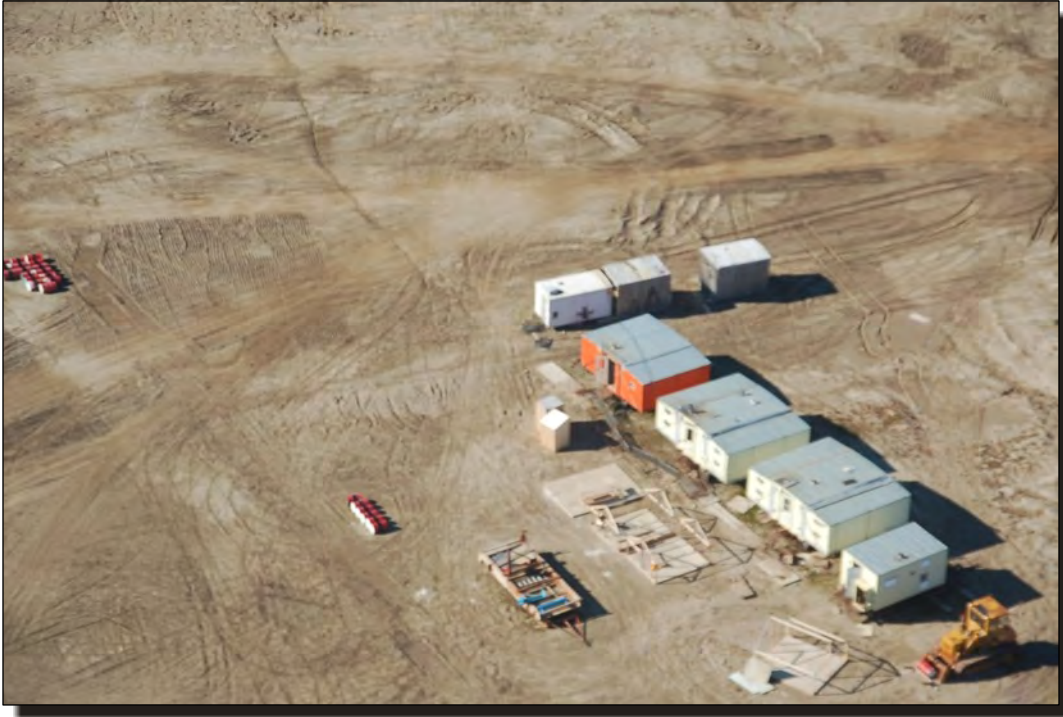
Photo 3 Close up aerial oblique of apron area.
