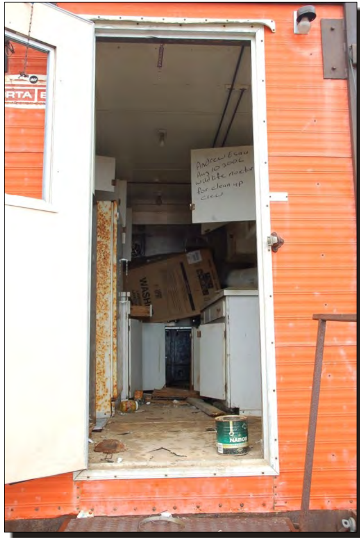
Photo 18 Interior of trailers at apron area.
