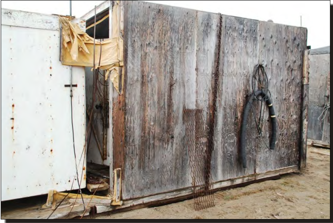
Photo 19 Shed at apron area.
