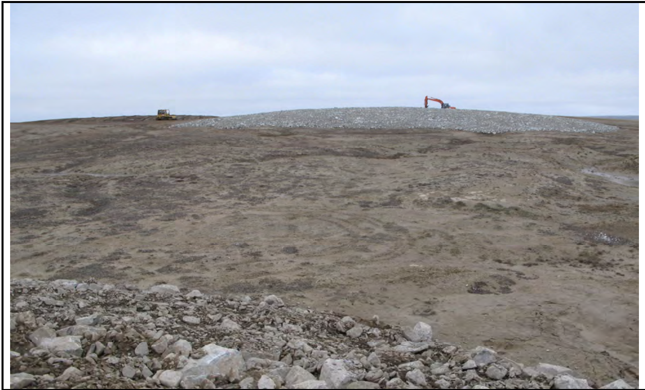
Photo 37: View from finished Landfill Regrade B towards finished Landfill Regrade C
