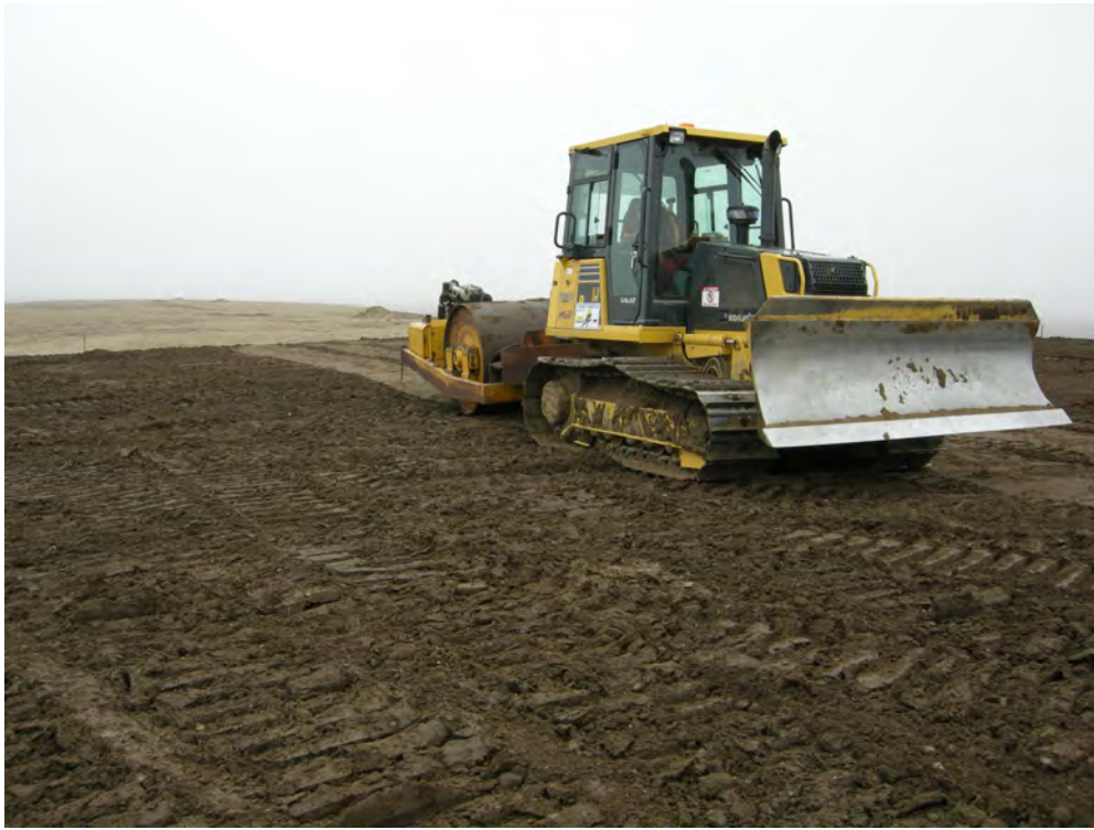
Photo 33: Vibration roller compaction of Type 2 material on Landfill Regrade D
