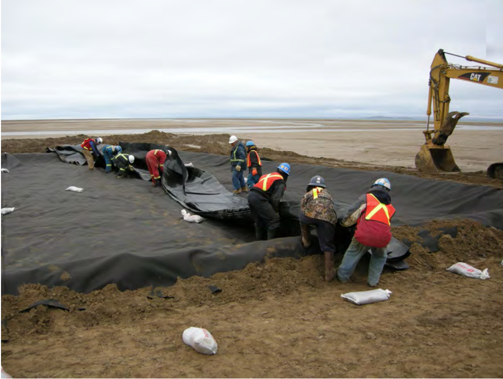
Photo 3: Constructing Post Treatment Greywater holding Pond
