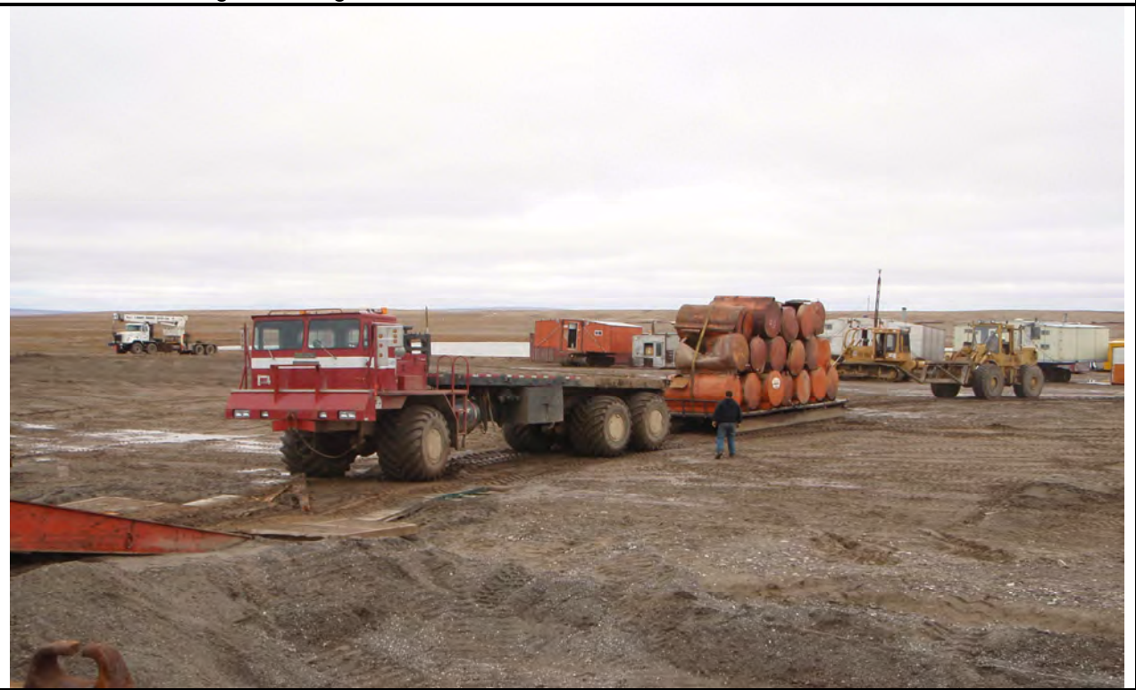
Photo 16: Loading non-hazardous waste on barge
