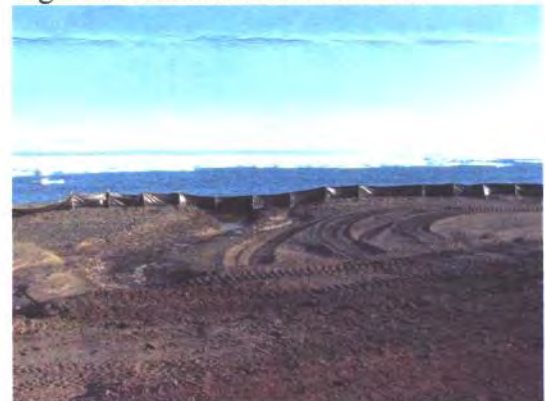
Figure 8: Sediment Containment
