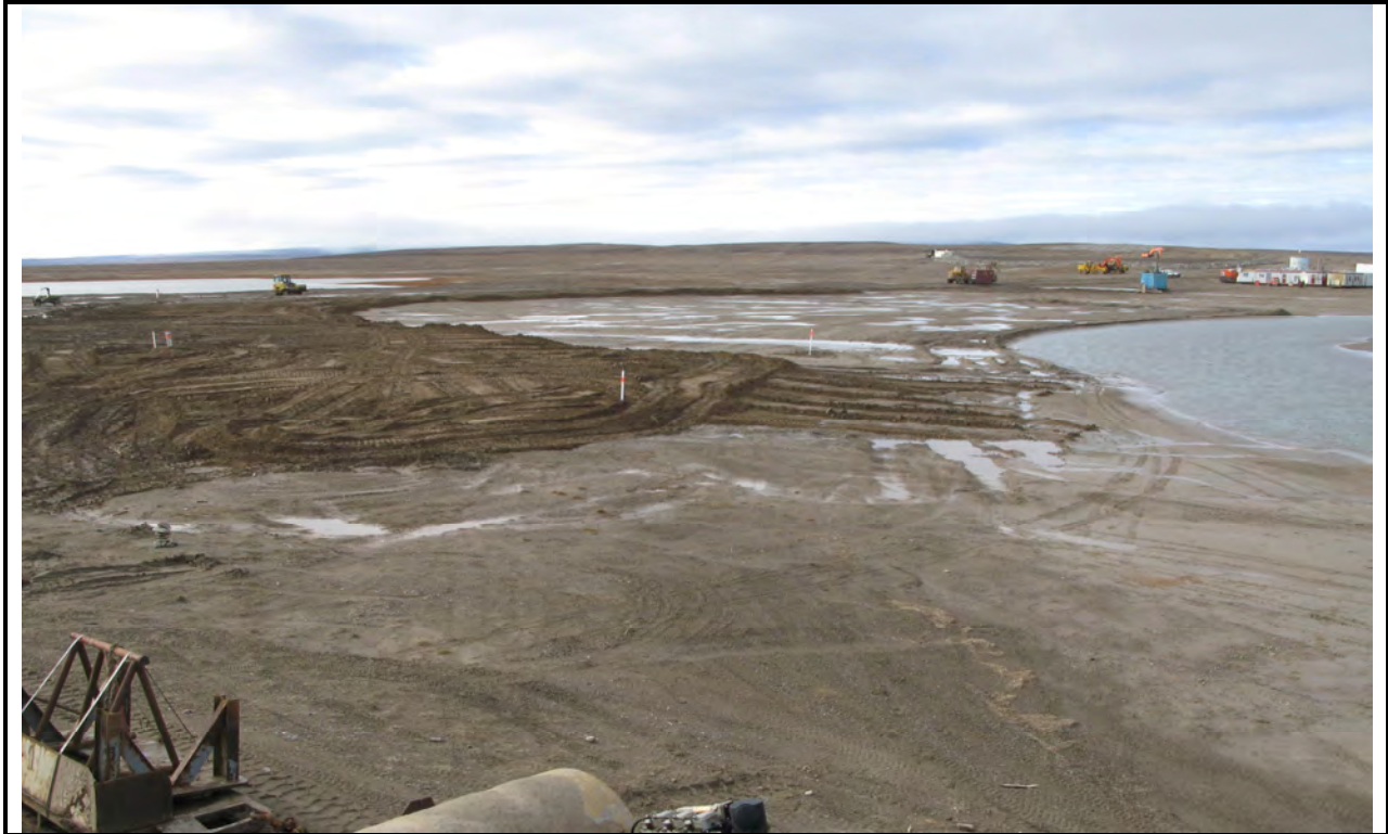
Photo 43: View west across backfilled Apron Area NE Plume
