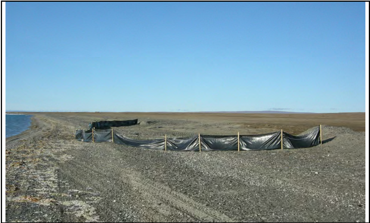
Photo 27: Silt screen erected around airstrip wash out during fill placement
