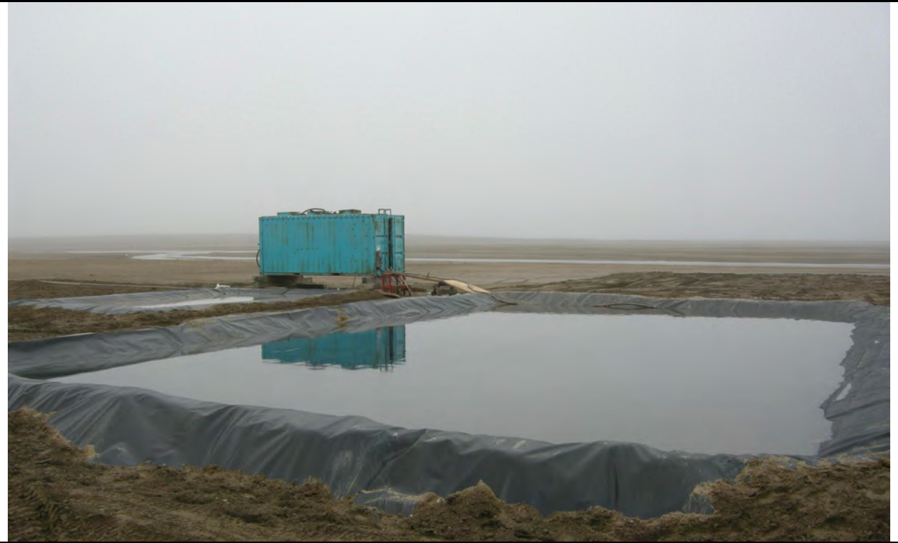
Photo 4: Greywater treatment system and holding ponds
