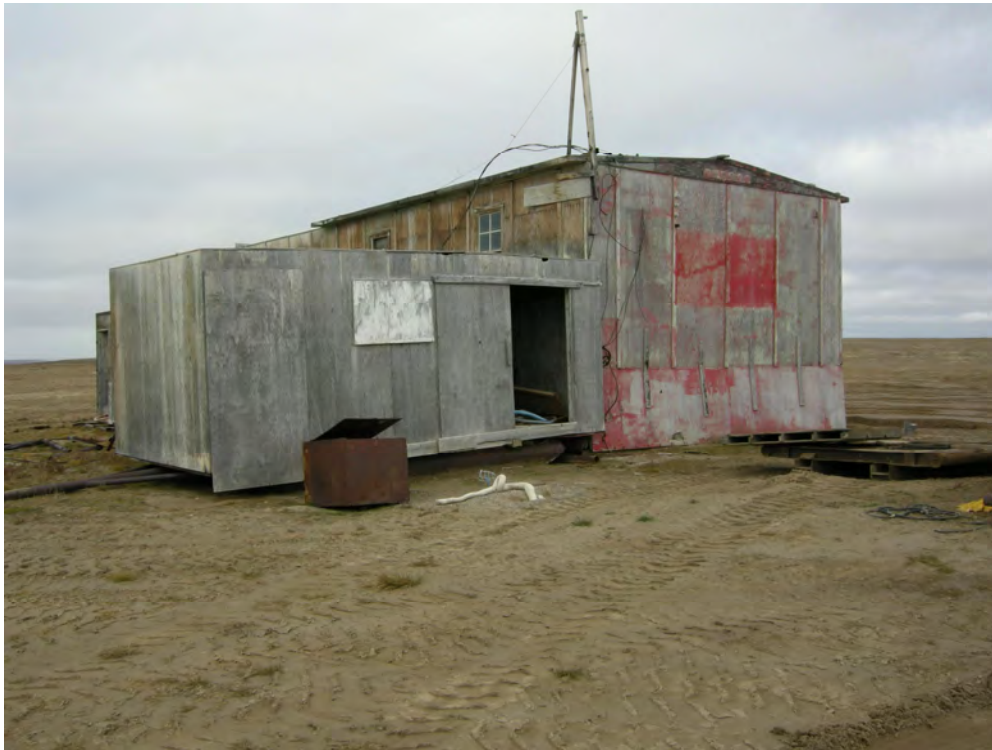
Photo 17: Main station maintenance building
