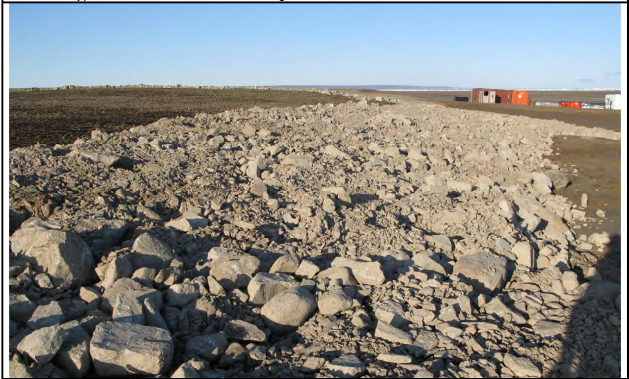
Photo 36: Type 1 material cover on SE slope of Landfill Regrade A
