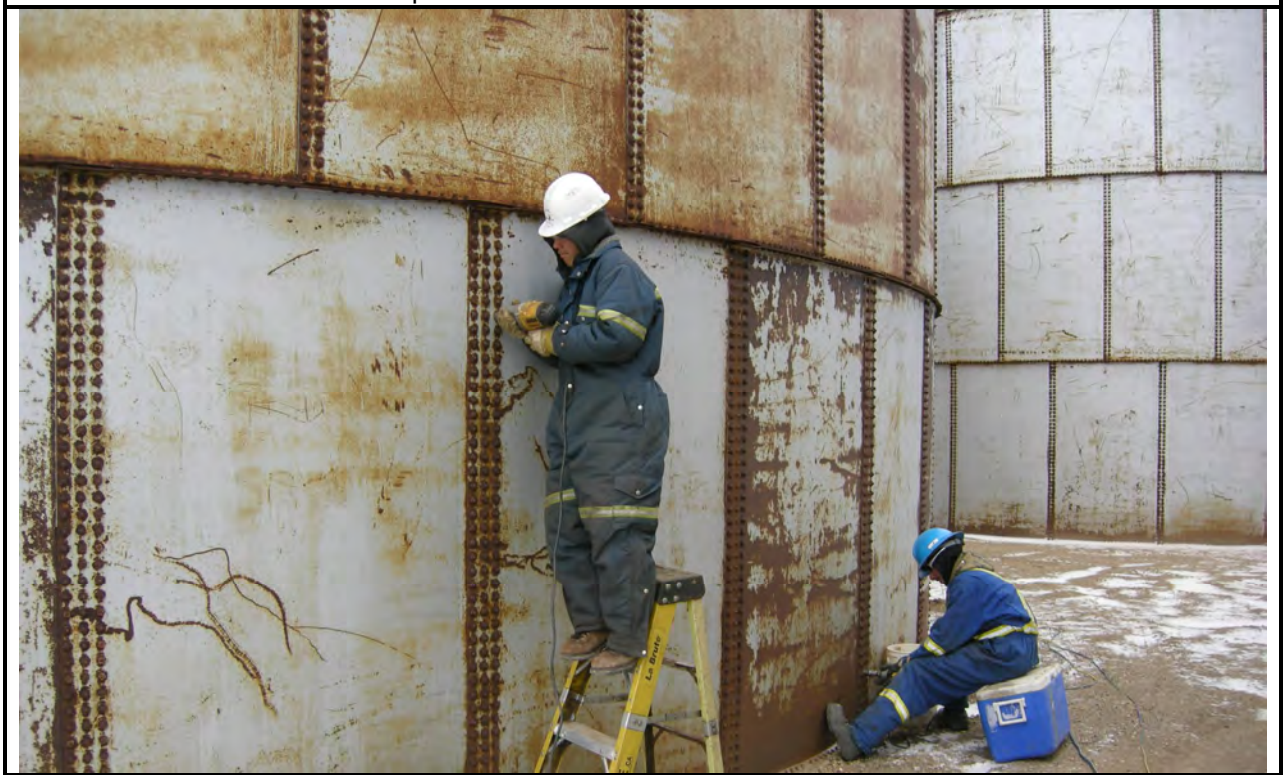
Photo 20: POL Tank demolition operations
