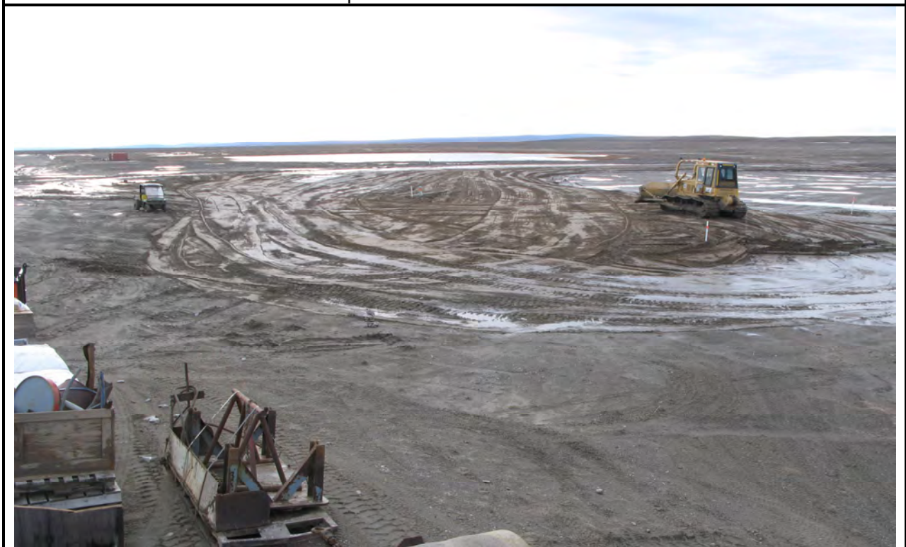
Photo 44: View SW across backfilled Apron Area excavations.
