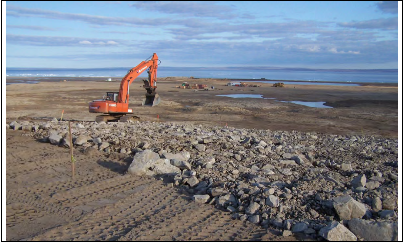
Photo 35: Type 1 material cover on Landfill Regrade C
