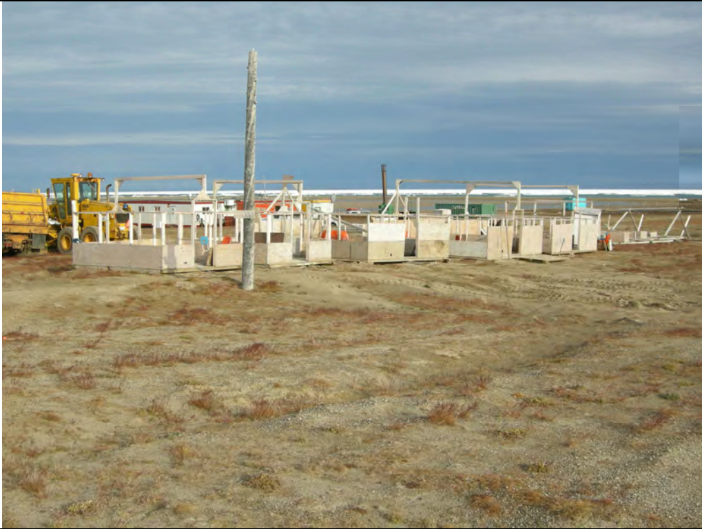
Photo 11: Wooden tent frames prior to demolition
