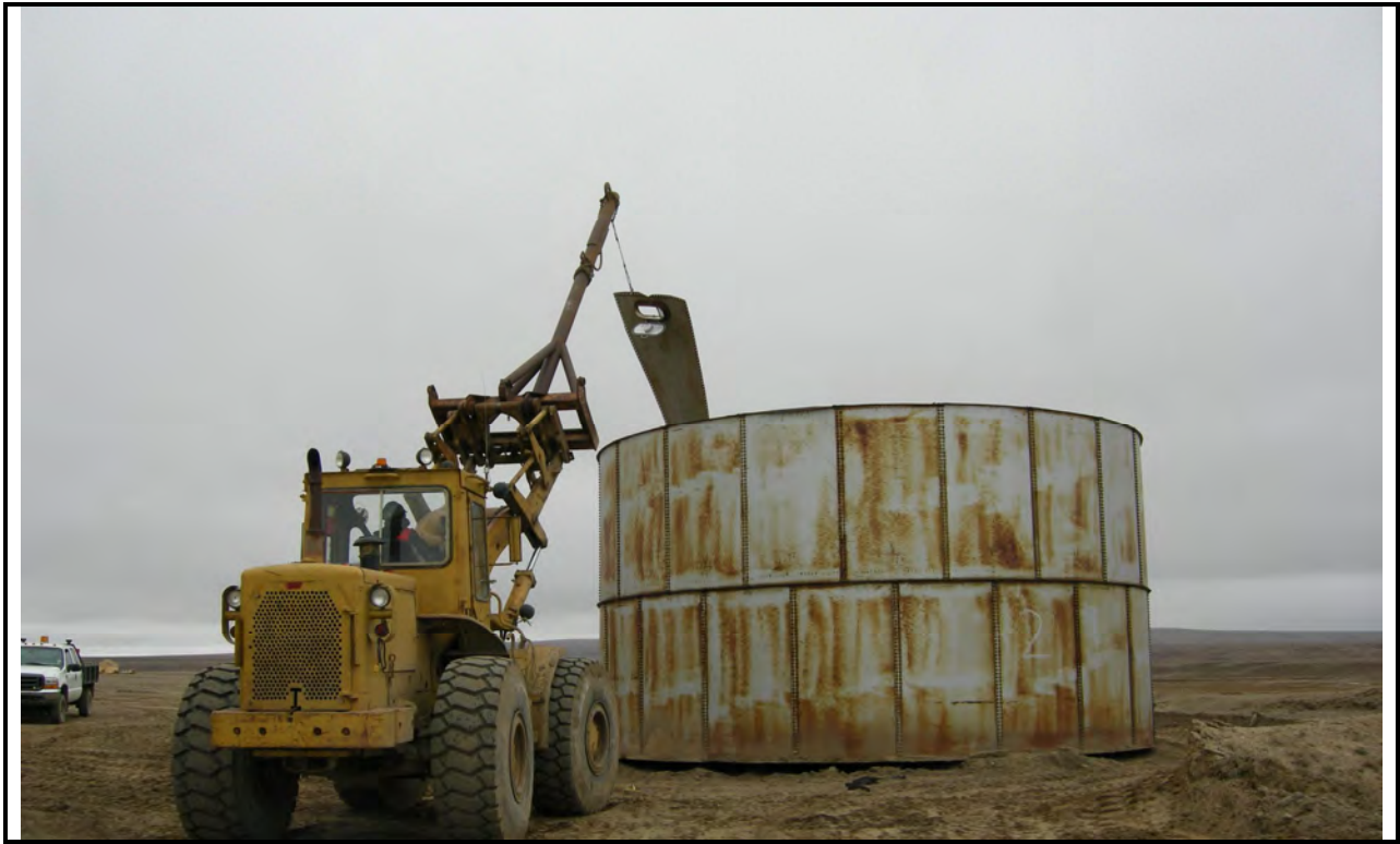
Photo 21: POL Tank demolition operations
