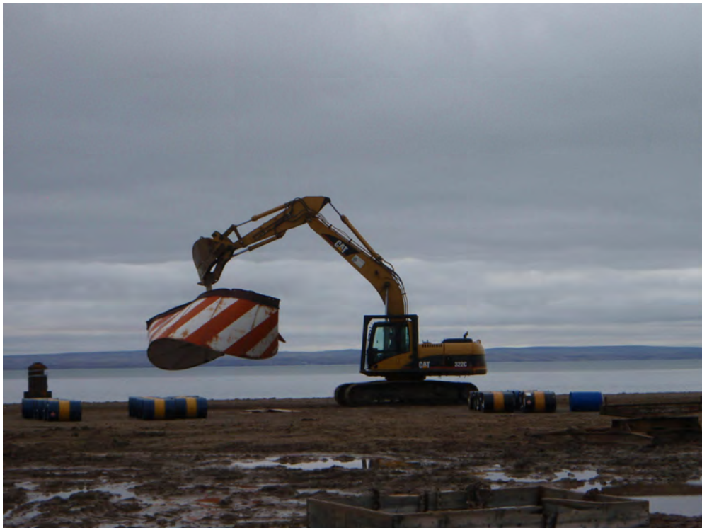
Photo 14: NAVAID structure during demolition
