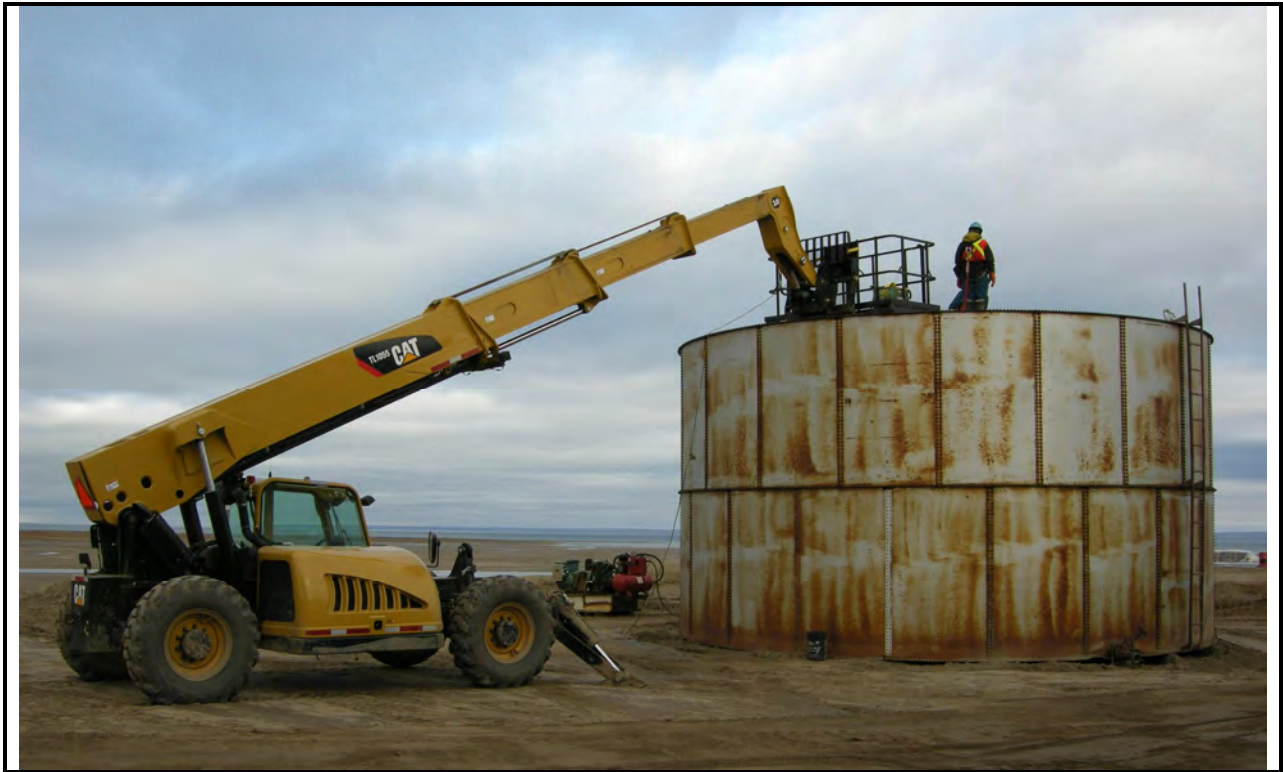
Photo 19: POL Tank demolition operations
