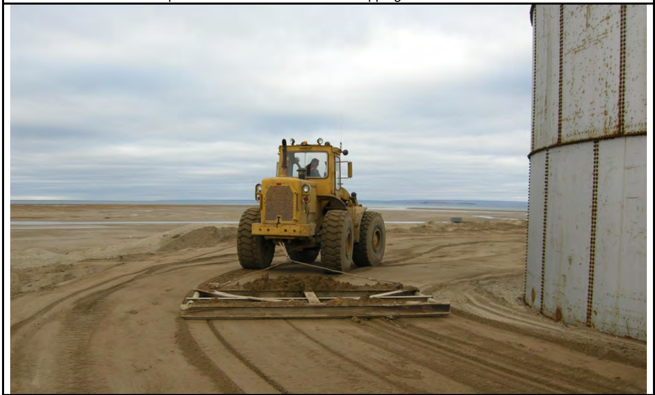
Photo 24: reshaping of tankfarm berms using drag
