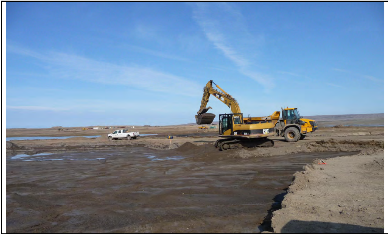
Photo 29: Excavation of Apron Area SW plume (Part 3)
