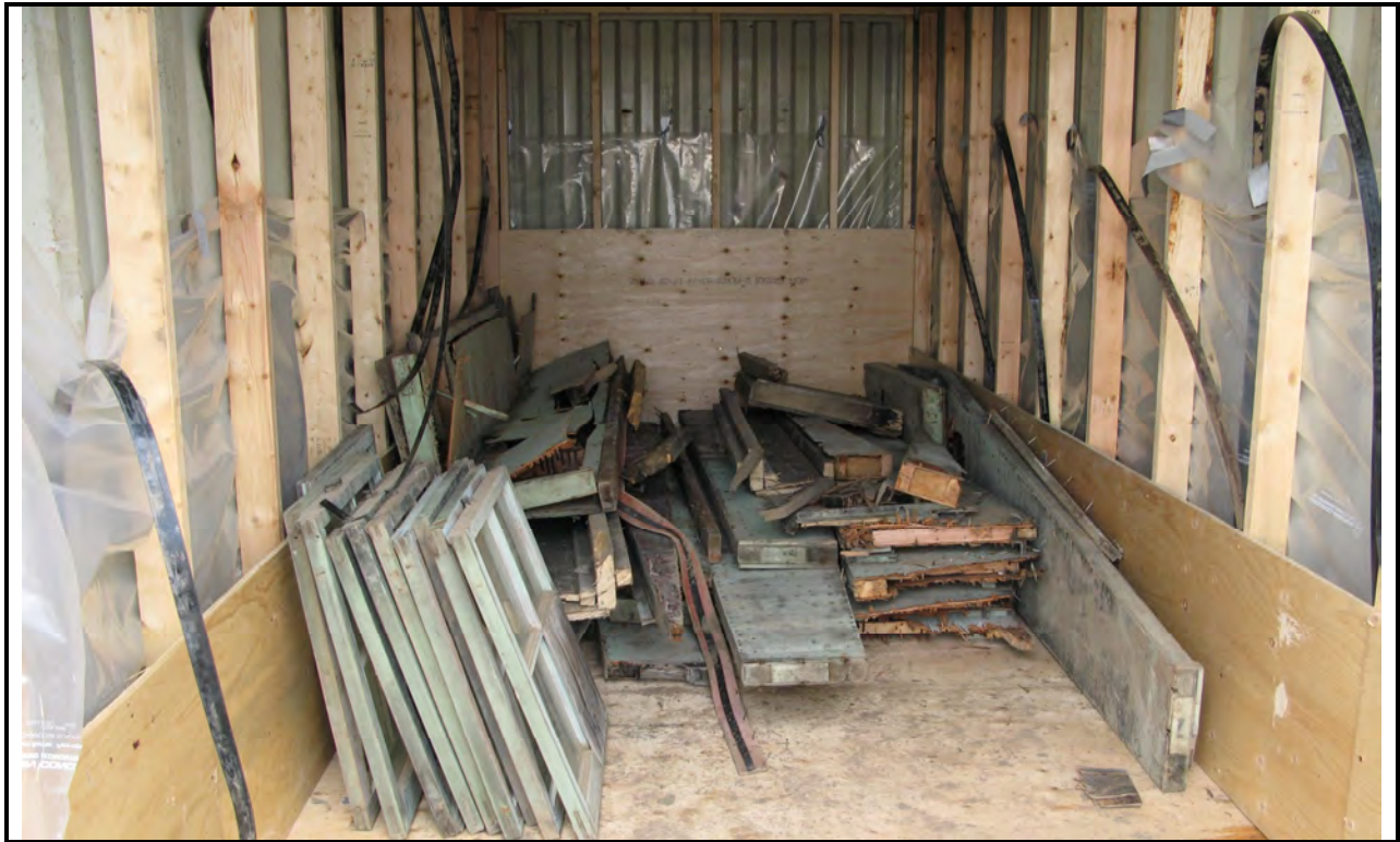
Photo 23: Leachable lead painted waste in lined Marine Shipping Container
