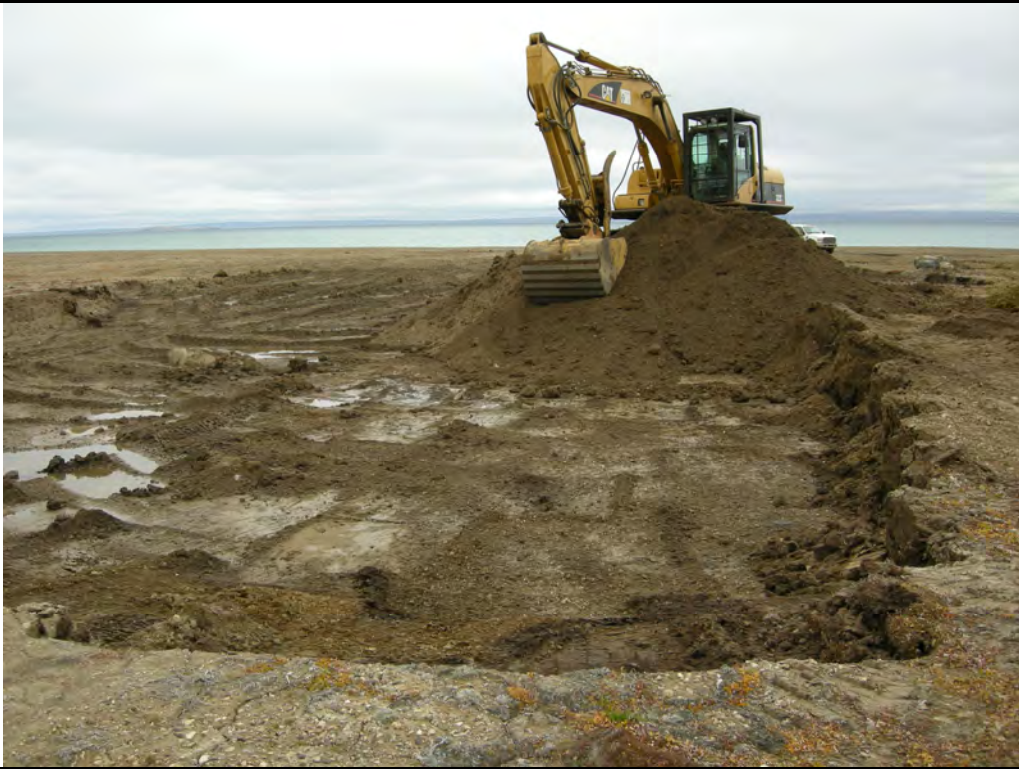
Photo 7: Initial stages of borrow extraction at Borrow Area B
