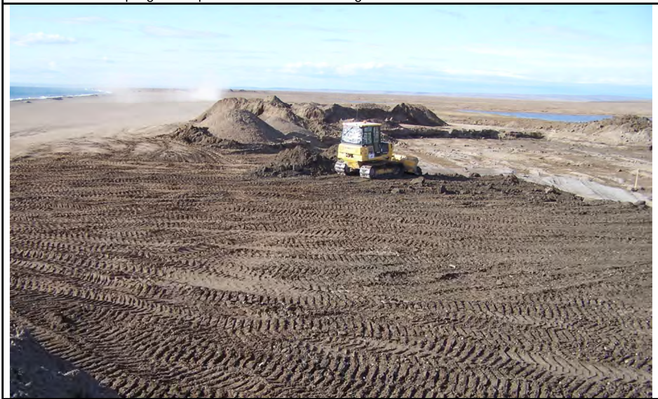
Photo 32: Trackpacking of SW Plume backfill material.
