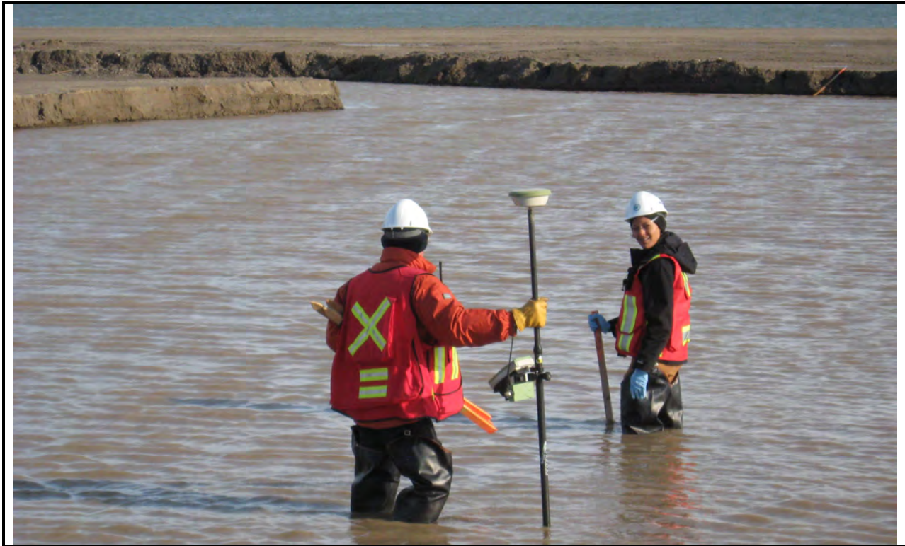
Photo 31: Soil sampling in SW plume excavation following rain
