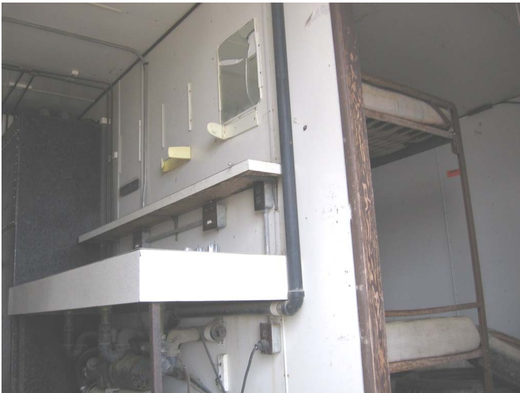
Photograph 20: Paint/Substrate Sample No. 7 White paint in Nodwell – Johnson Point 2007
