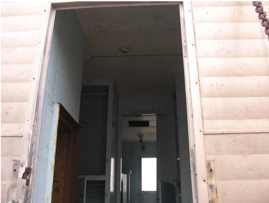
Photograph 18: Paint/Substrate Sample 4, from interior blue paint – Nodwells – Johnson Point 2007
