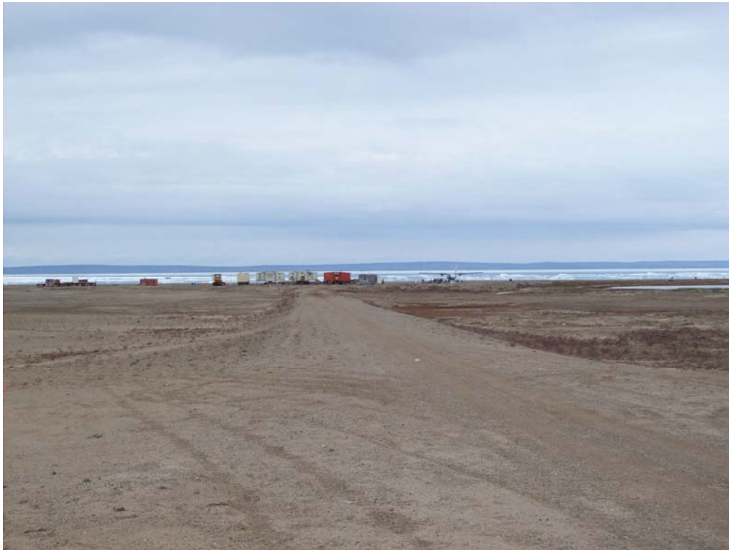
Photograph 5: View along access road towards apron – Johnson Point, 2007
