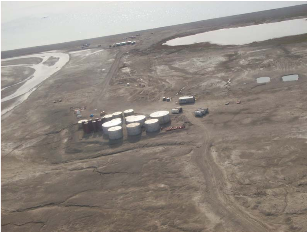
Photograph 2: Aerial View of Site from Tank Farm towards Apron – Apron Pond to right - Johnson Point 2007
