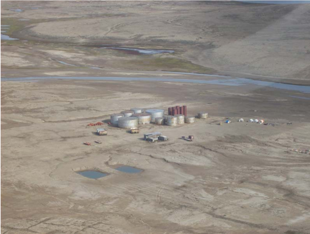
Photograph 3: Aerial View of Tank Farm – Johnson Point 2007.
