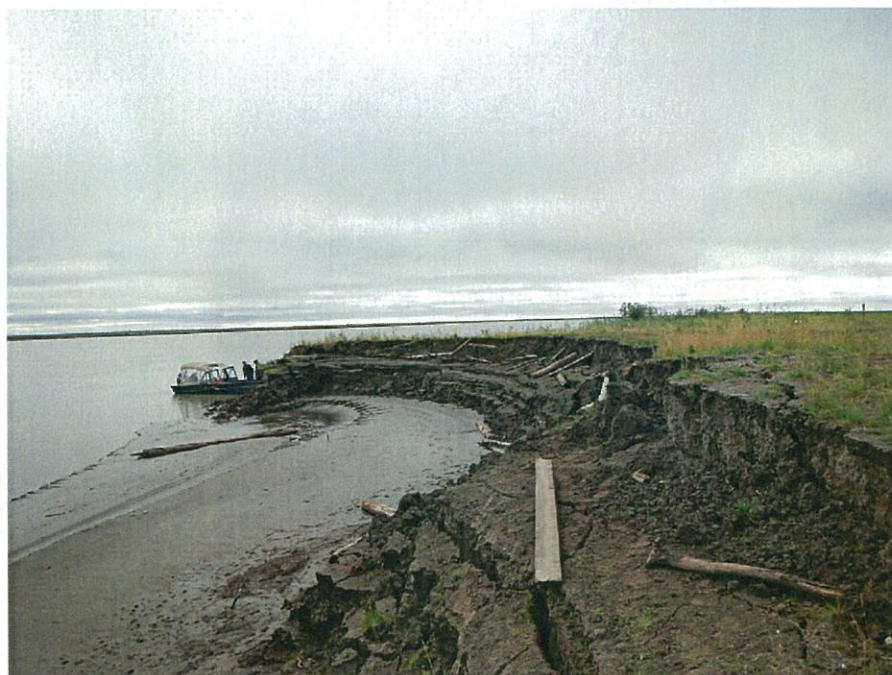
Photograph 3: View southwest of timber debris placed on eroded riverbank (August 17, 2013).
