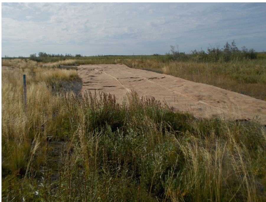
Photograph 10: Coconut matting staked down over area of sparse vegetation on northern portion of the backfill cap (August 12, 2014).
