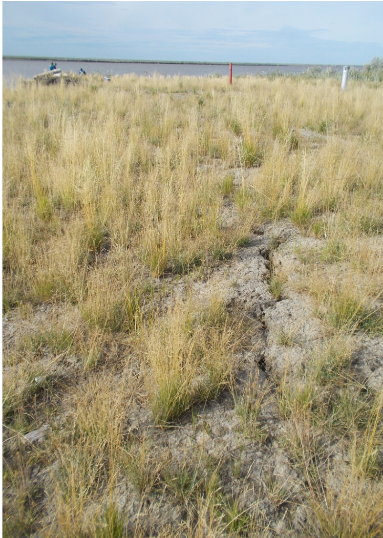
Photograph 3: Vegetation establishing on backfill cap. Cracks observed approximately 10 m back from the bank (August 12, 2014).
