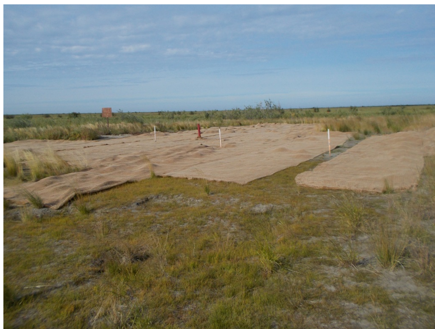
Photograph 7: Coconut matting staked down over area of sparse vegetation west of the backfill cap (August 12, 2014).
