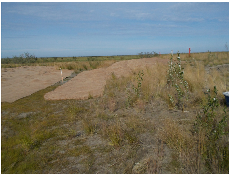
Photograph 8: Coconut matting staked down over area of sparse vegetation on western portion of the backfill cap (August 12, 2014).
