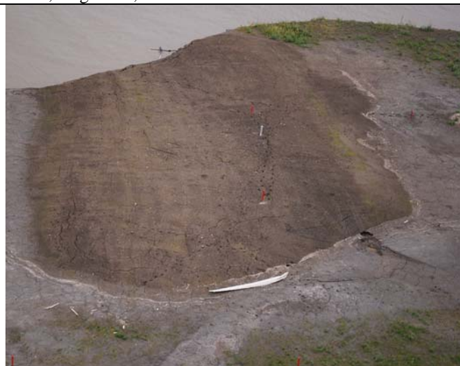
Figure 6 Sump backfill area with erosion of southeast corner. Subsidence and what appears to be a sink hole on the northwest corner of the former sump area, August 24, 2011.
