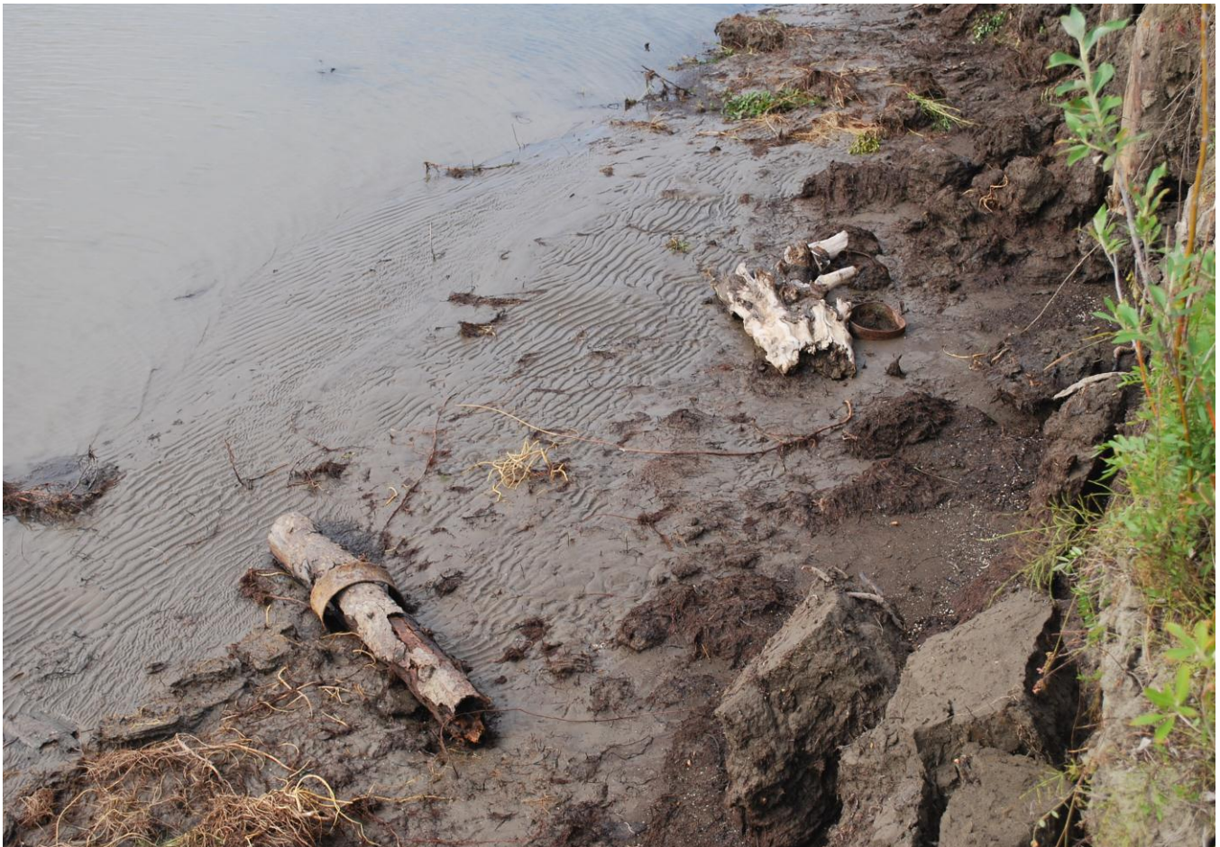
Figure 4 cut pipe on pilings
