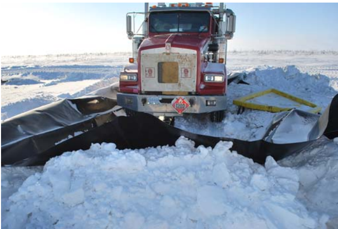
Figure 5 Main tanker truck fuel storage area - bermed with synthetic liner.
