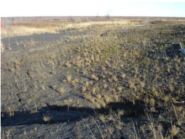
Figure 5 Erosion channel that exists on site. Continued monitoring is needed to mitigate possible risks to site stability by increased erosion, October 2, 2012.
