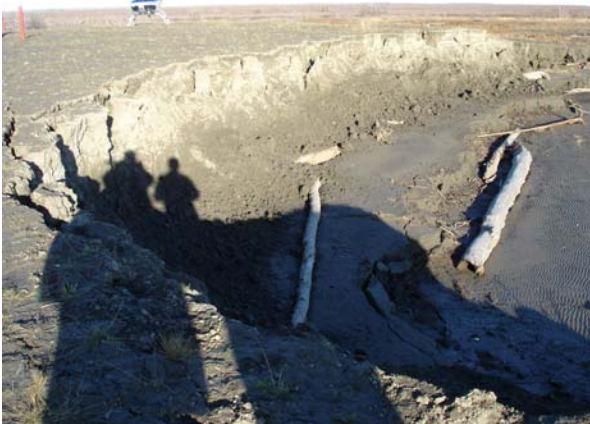
Figure 3 Close up of erosion and further river embankment that has been washed away, October 2, 2012.
