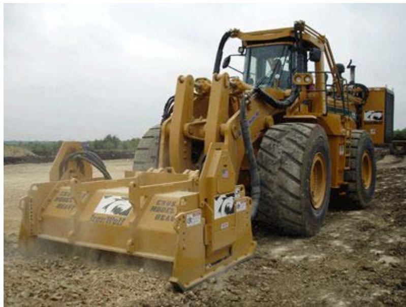
Photo 5-1: Proposed IronWolf™ Excavation Method
