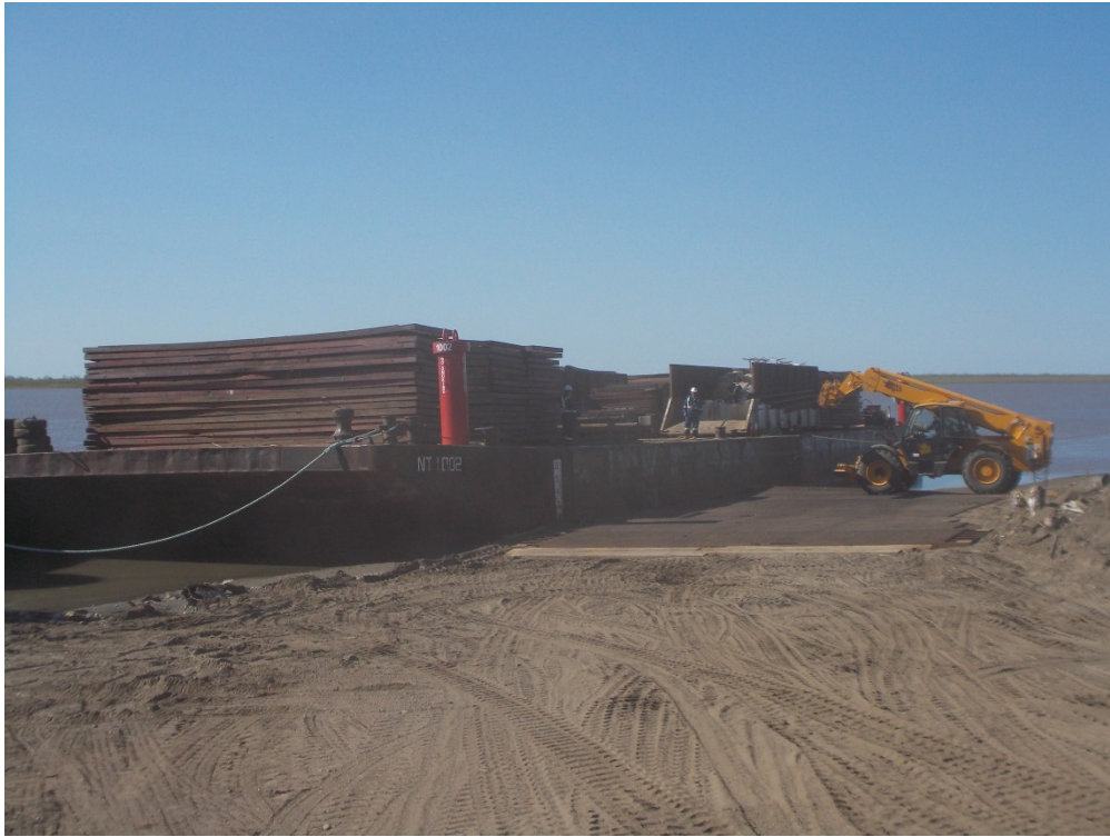
Photograph 11: Rig mats laid down on river shore for equipment to load barges (August 11, 2014).
