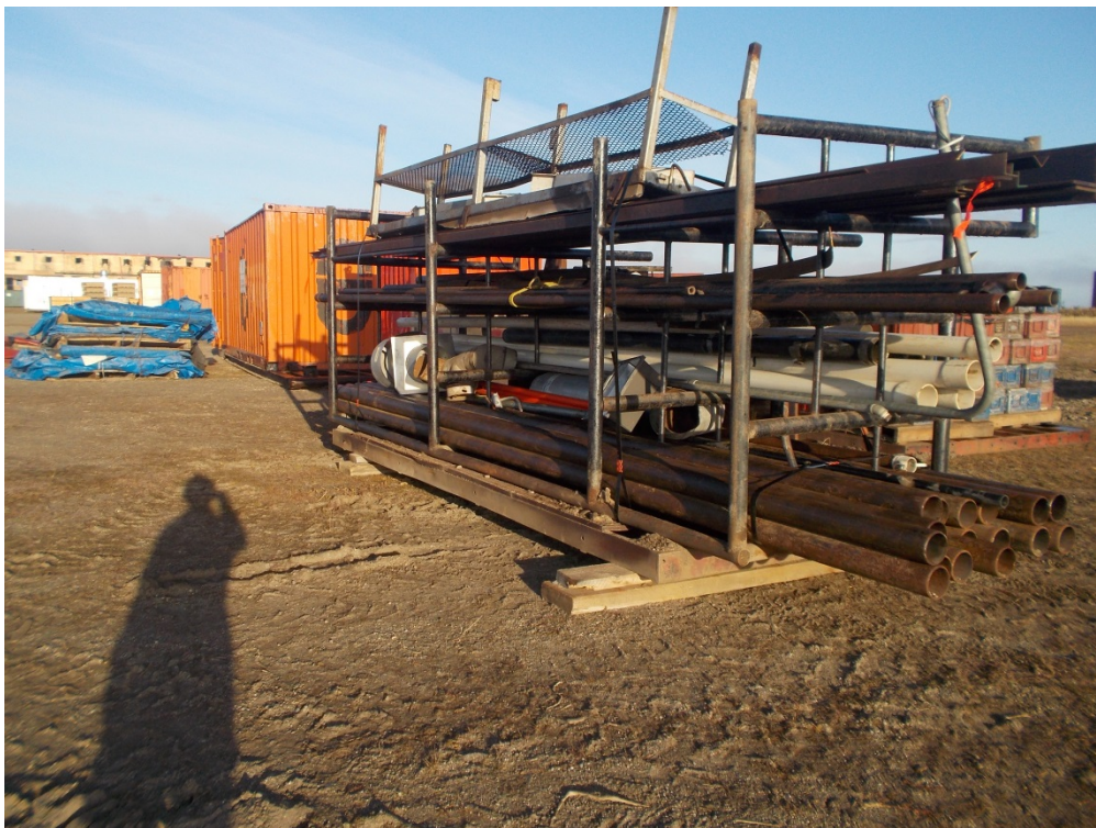
Photograph 8: Materials to be removed from Site (August 19, 2014).
