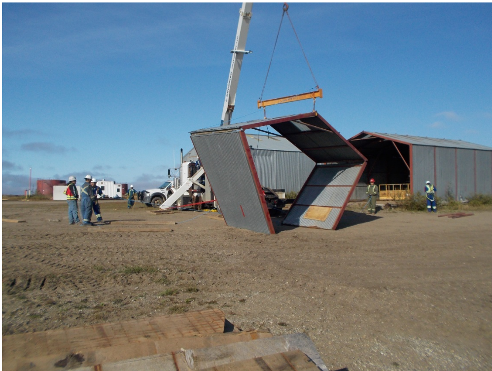
Photograph 2: Disassembly of Shed #2 (August 19, 2014).
