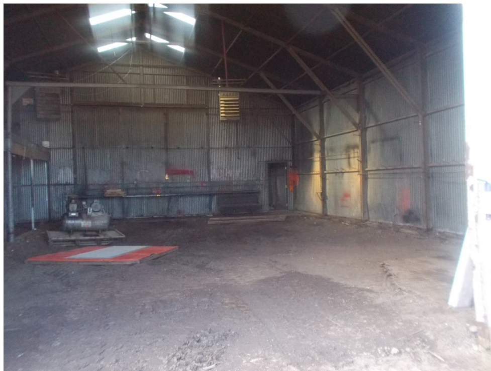
Photograph 14: Dirt floor of Shed #1 where composite soil samples were collected (August 17, 2014).
