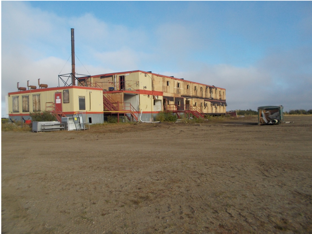
Photograph 1: Camp building in the process of decommissioning (August 19, 2014).
