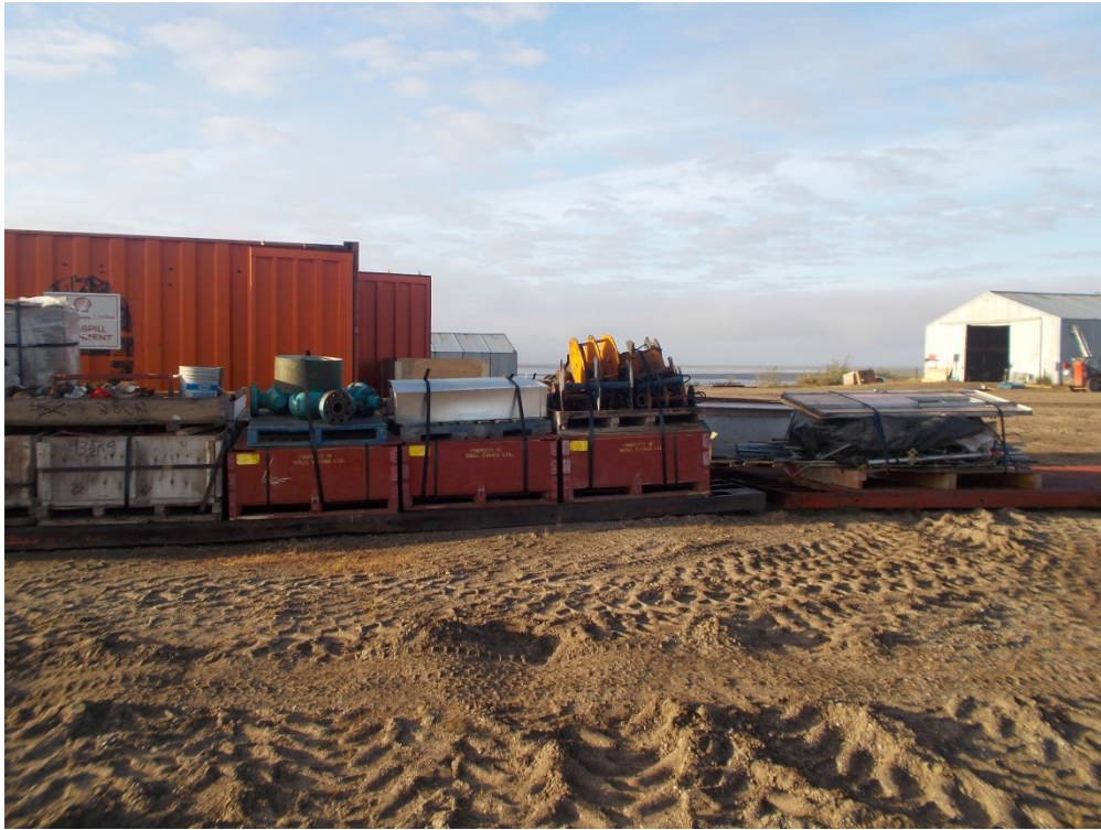
Photograph 9: Materials to be removed from Site (August 9, 2014).
