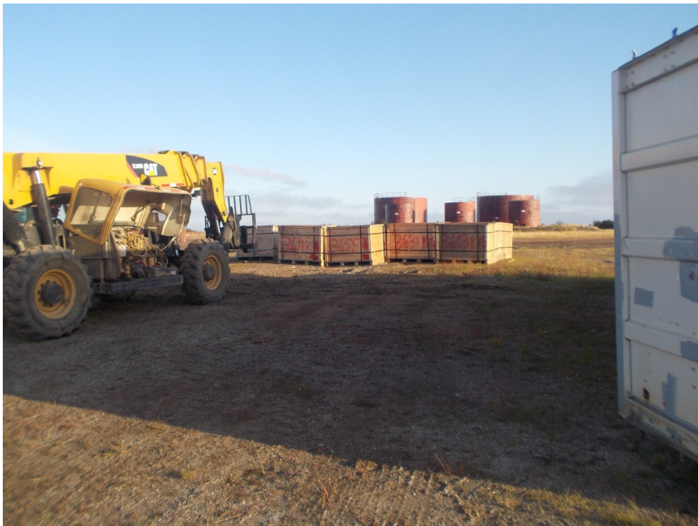
Photograph 10: Wooden crates for transporting materials (August 19, 2014).
