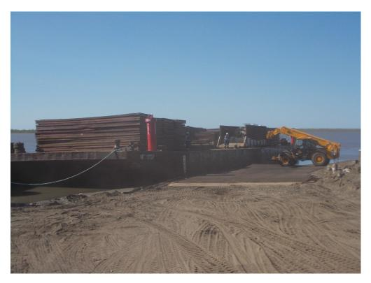
Photograph 11: Rig mats laid down on river shore for equipment to load barges (August 11, 2014).
