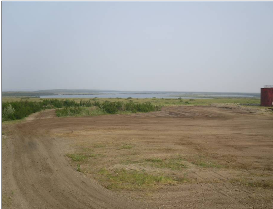
Photograph 8: Excavation #1 following backfilling.
