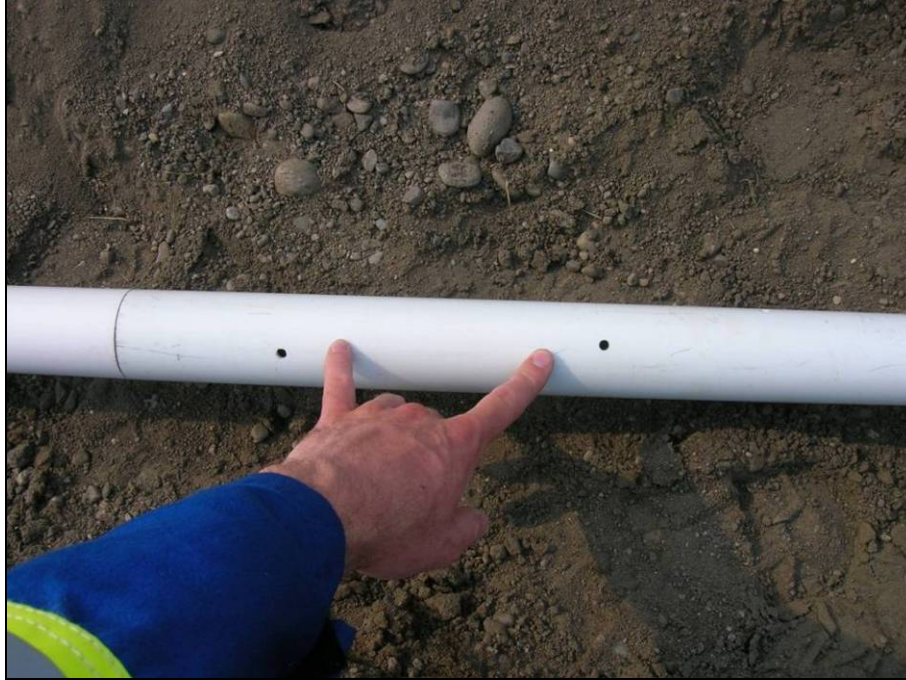
Photograph 7: Perforations made on-site. Holes are spaced around all sides of the pipe.
