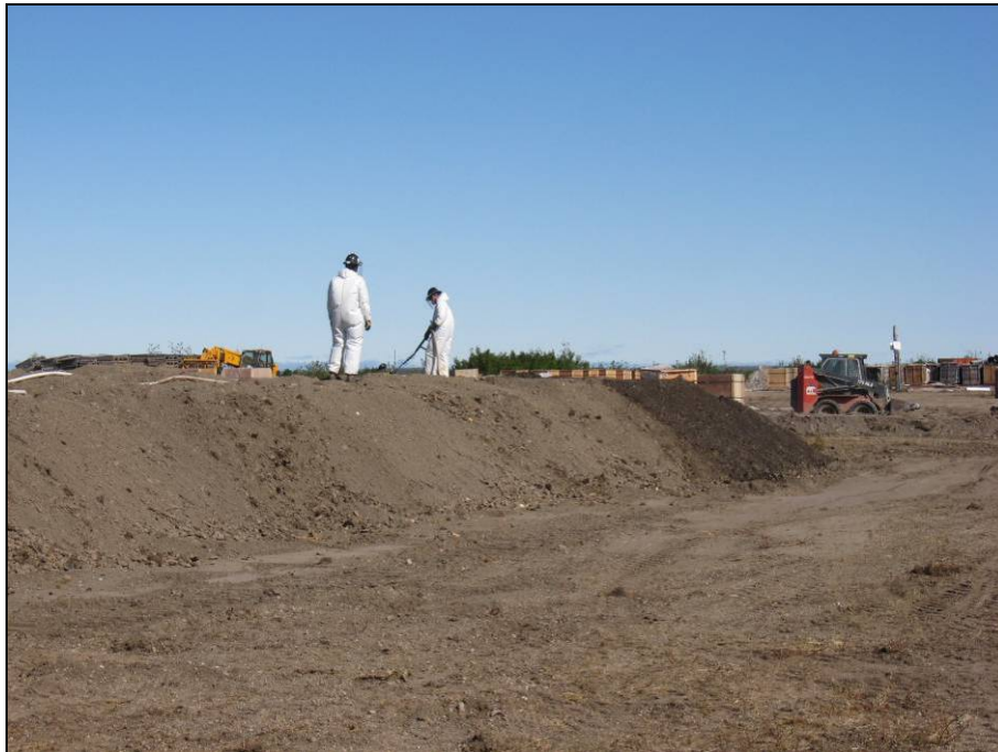
Photograph 2: RegenOx (Part B) being applied to a windrow
