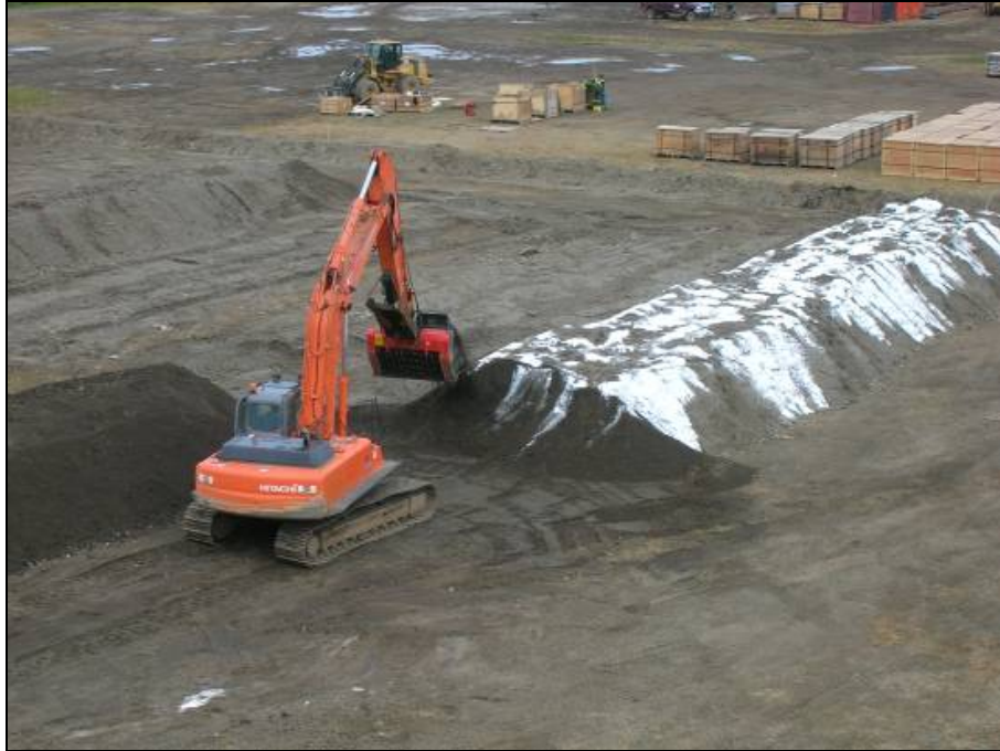
Photograph 3: RegenOx (Part A) being mixed into windrow 3.
