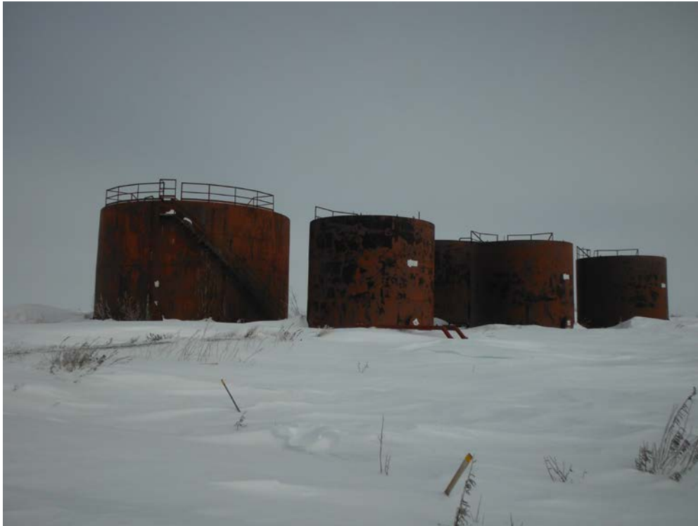
Photograph 1: Snow covered conditions and storage tanks in good condition (April 27, 2013).
