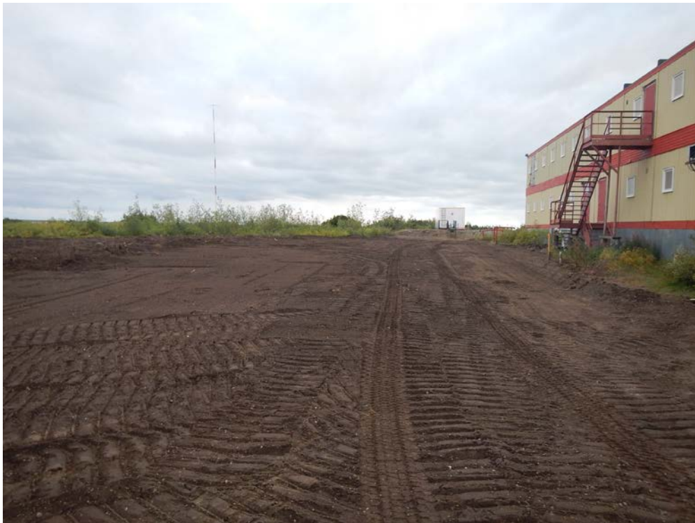
Photograph 8: Remediated and backfilled lagoon and camp building in good condition (August 25, 2013).
