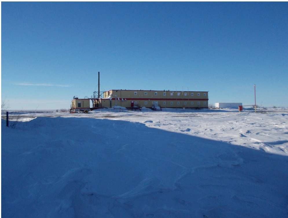
Photograph 4: Camp building and snow covered ground conditions (March 13, 2014).
