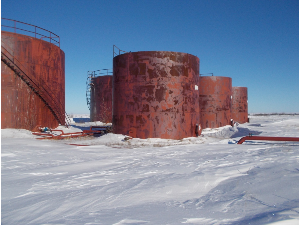
Photograph 3: Tank farm in good condition (March 13, 2014).
