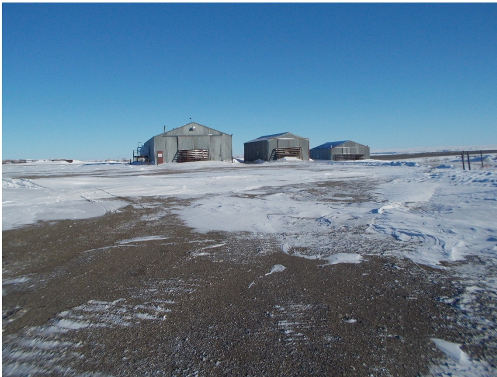
Photograph 2: : Snow covered ground conditions and buildings in good condition (March 13, 2014).
