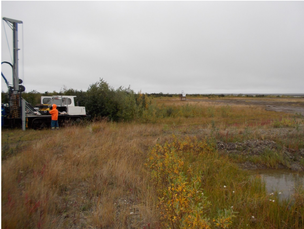
Photograph 3: View northwest of laydown area and drilling activities (August 18, 2015).
