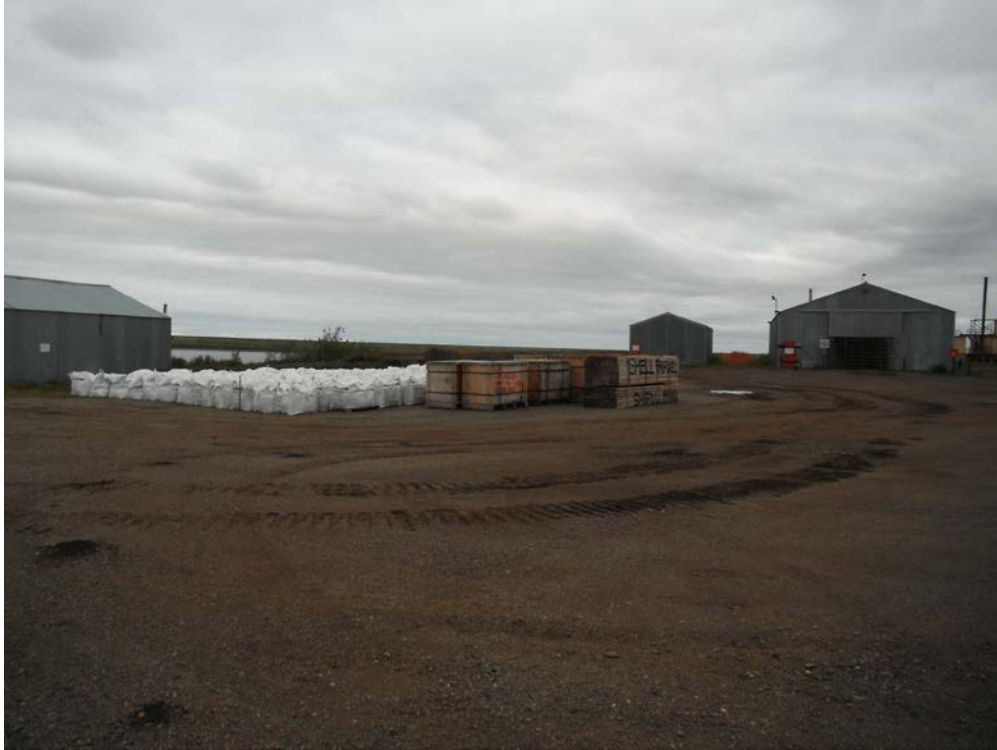
Photograph 7: View of soil bag staging area and buildings in good condition (August 25, 2013).
