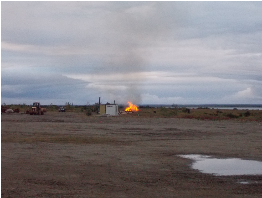
Photograph 4: View east of emergency shelter and decommissioning activities (August 18, 2014).
