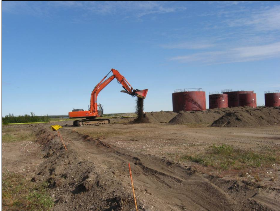
Photograph 1: Impacted soils being aerated with an allu bucket inside the treatment cell.
