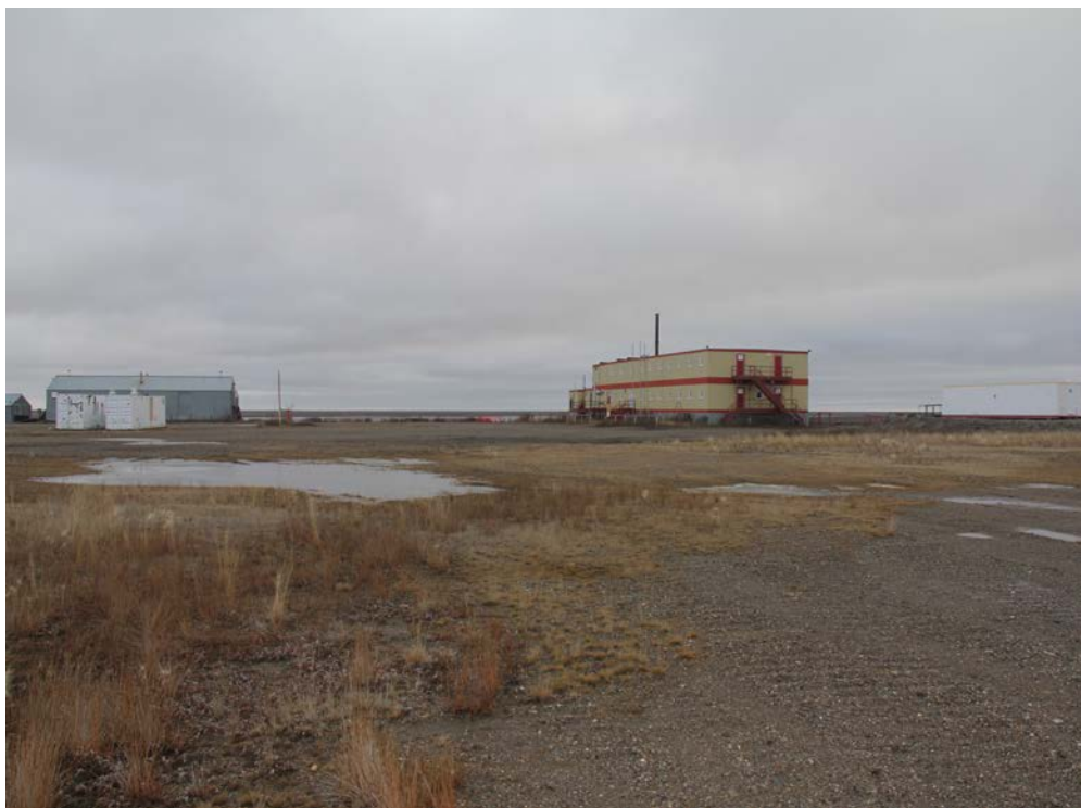
Photograph 10: Buildings in good condition at Camp Farewell (October 9, 2013).
