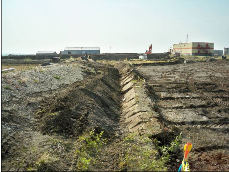
Photograph 5: In situ subsurface treatment trench looking south.
