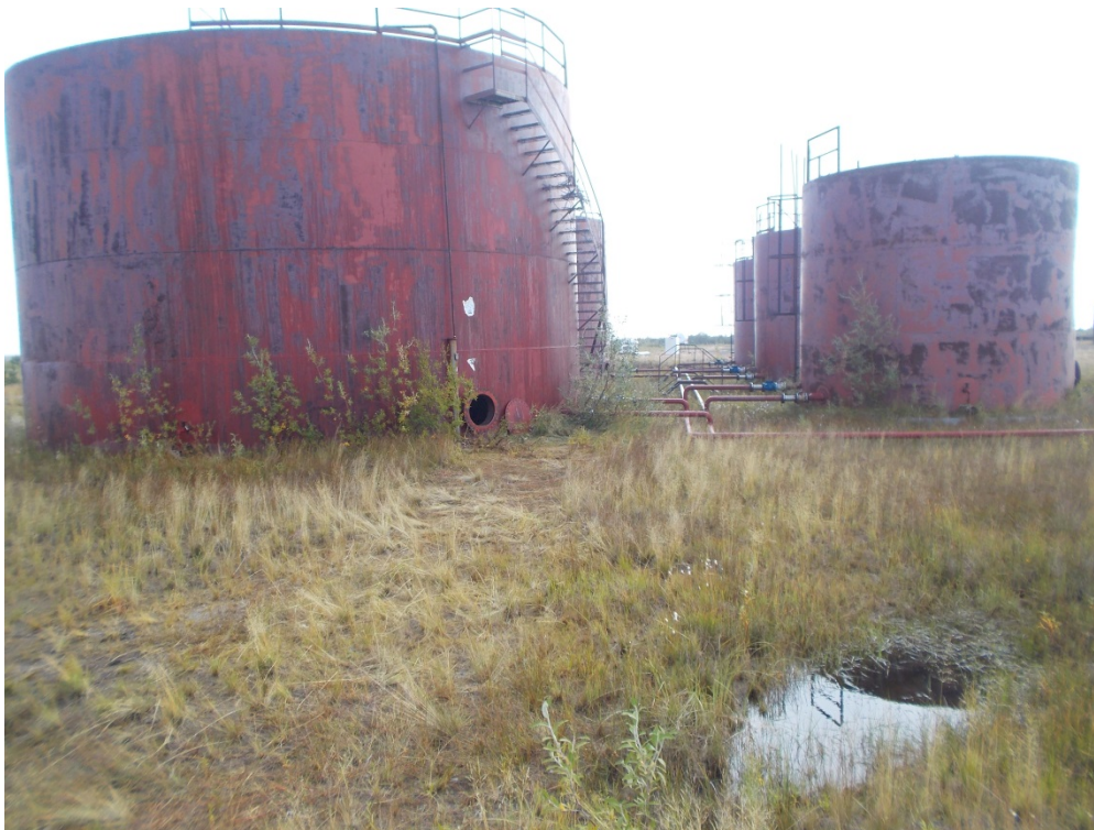
Photograph 8: View of tank farm (August 19, 2014).
