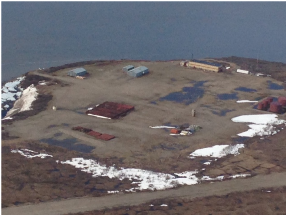
Photograph 6: Aerial view of Camp Farewell (June 12, 2013).
