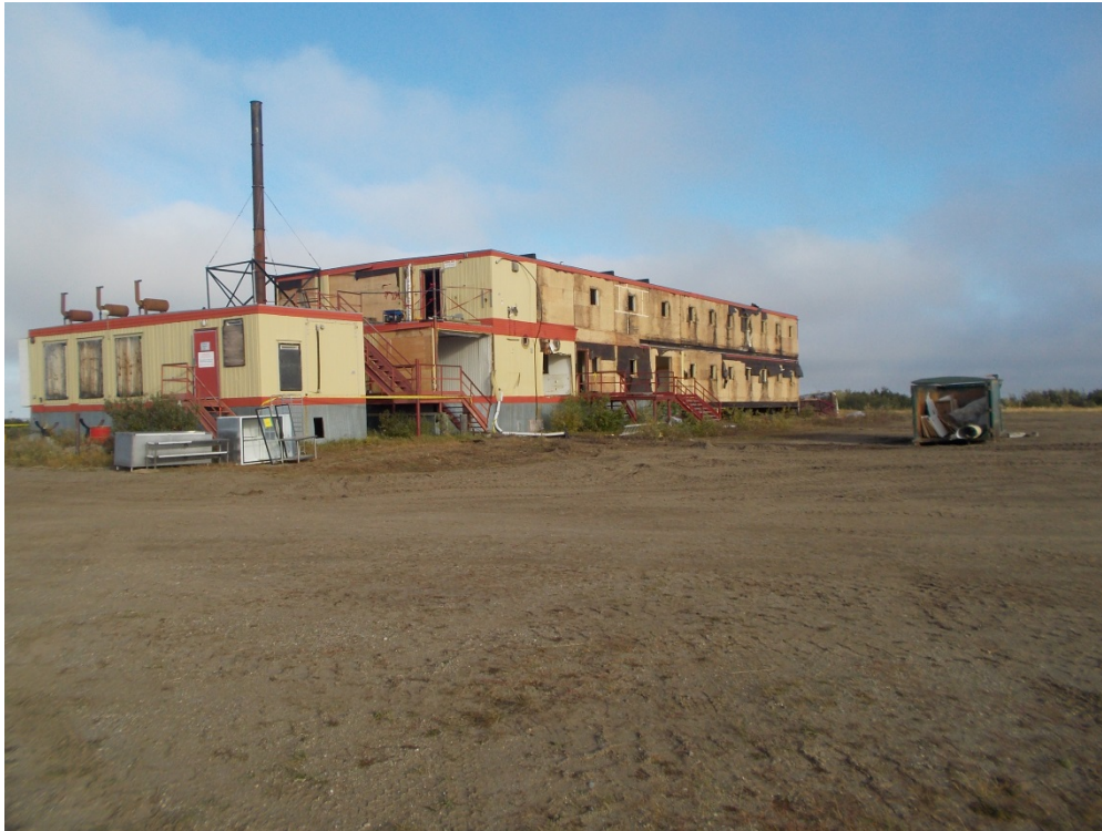
Photograph 5: Camp building in the process of being taken down (August 19, 2014).
