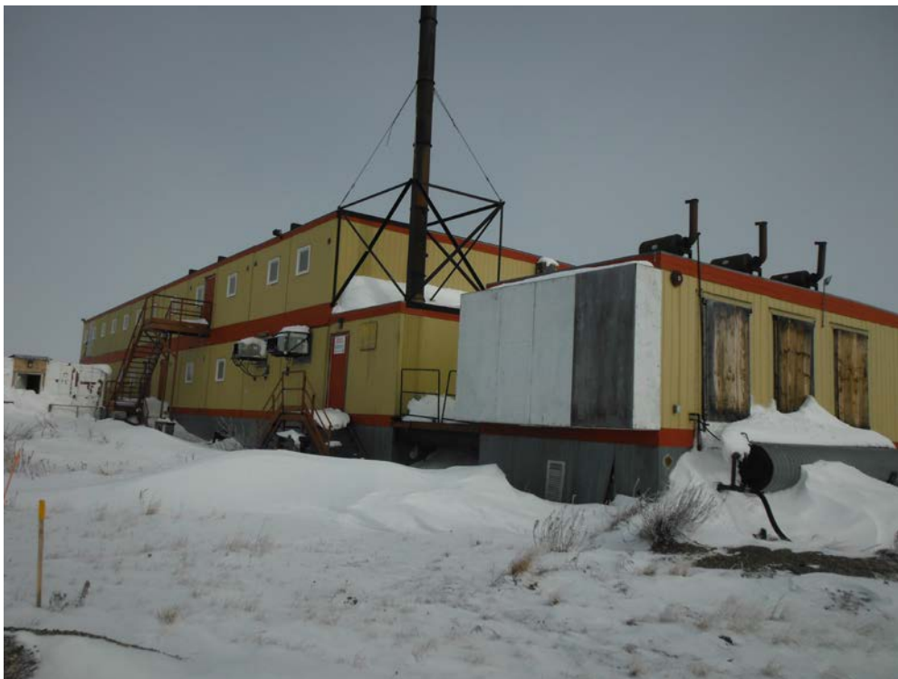
Photograph 2: Snow covered conditions and buildings in good condition (April 27, 2013).
