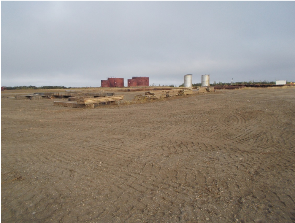
Photograph 7: View of Site, facing northwest (August 19, 2014).
