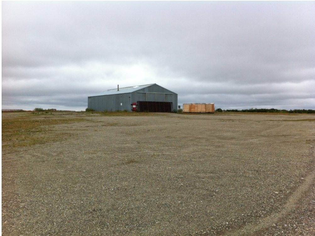
Photograph 1: View northwest of Shed #1 (August 11, 2015).
