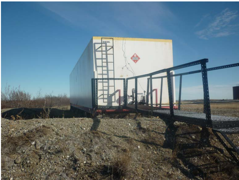
Photograph 4: Diesel storage tank in good condition (June 12, 2013).
