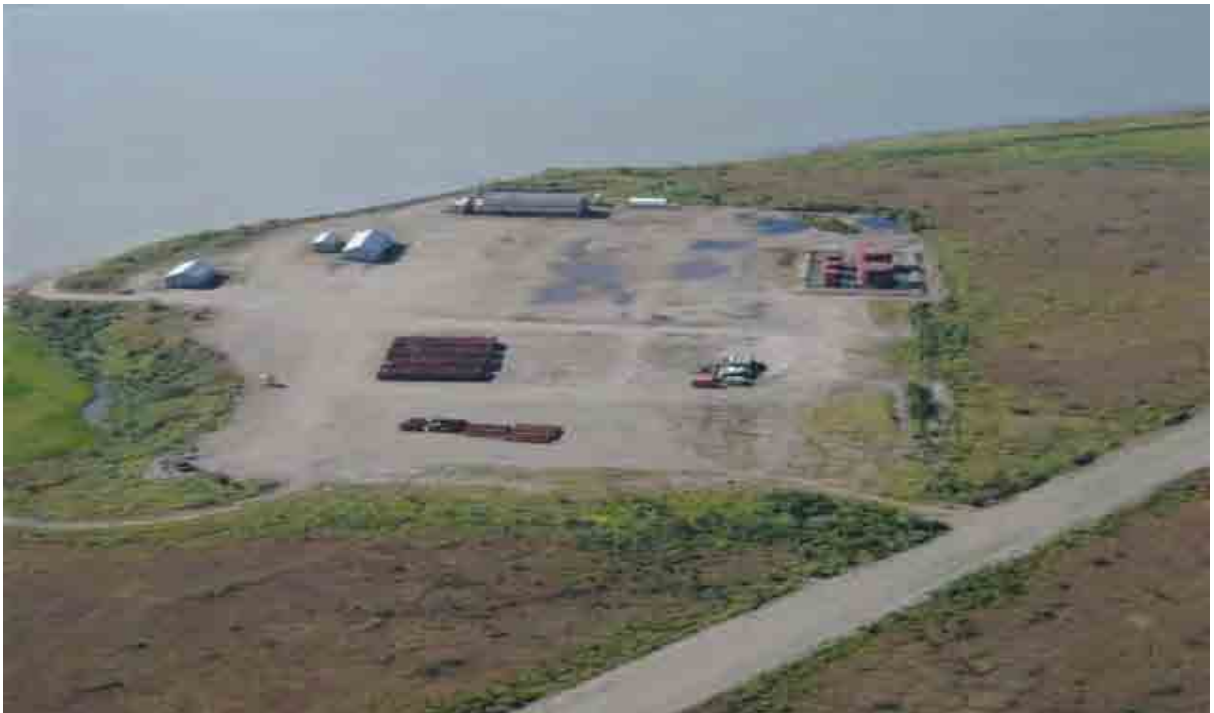
Photo 1: Aerial View of Stained and Pond Area (August, 2009)
