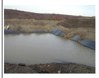
October – Water from the corner of the treatment cell was discharged before freezing.
