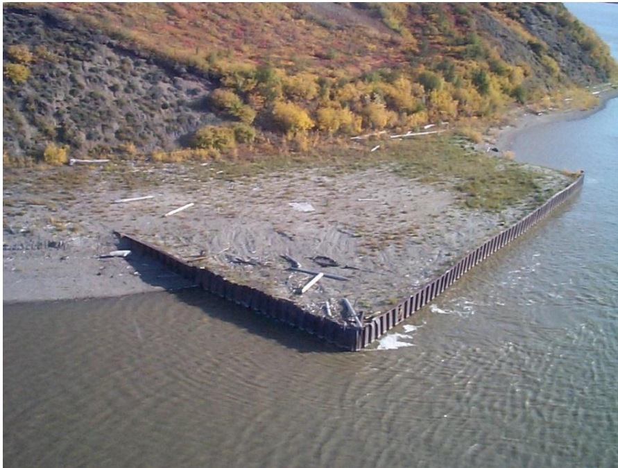
Photo 4: Aerial view of the dock
