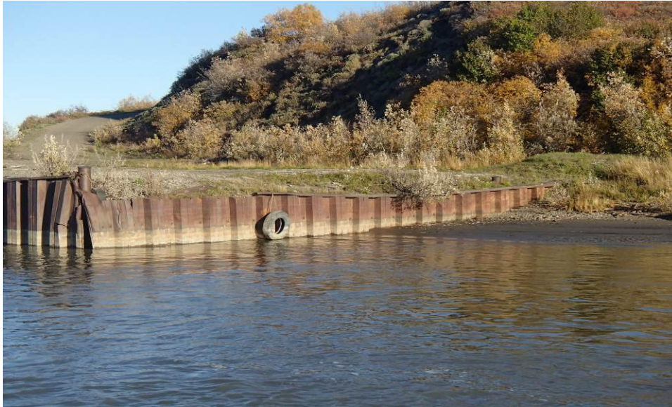
Photo 3: General view of the east wall.
