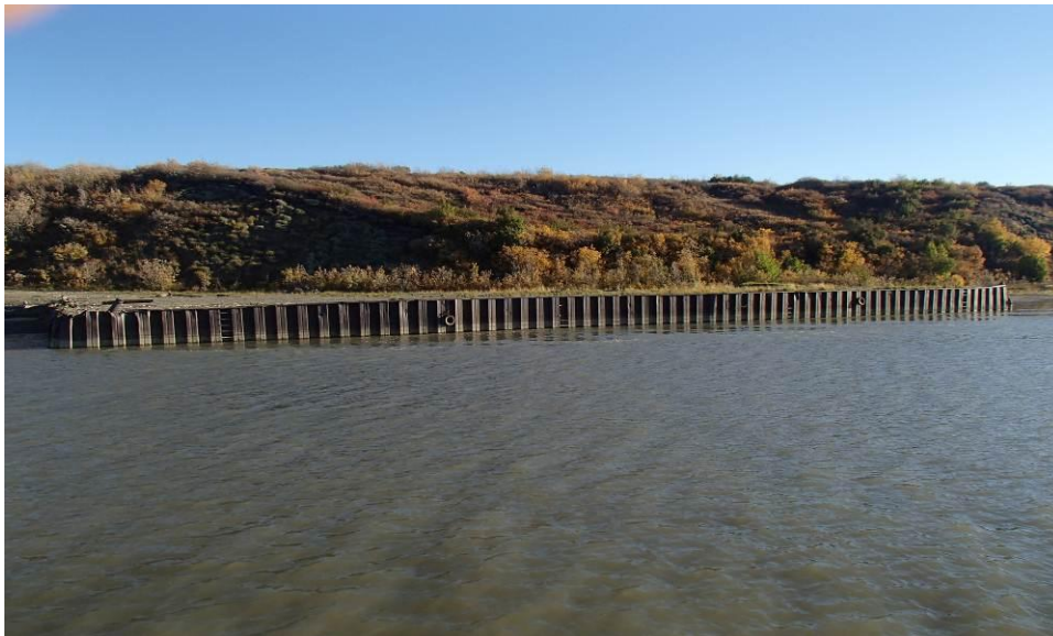
Photo 2: General view of the south wall.
