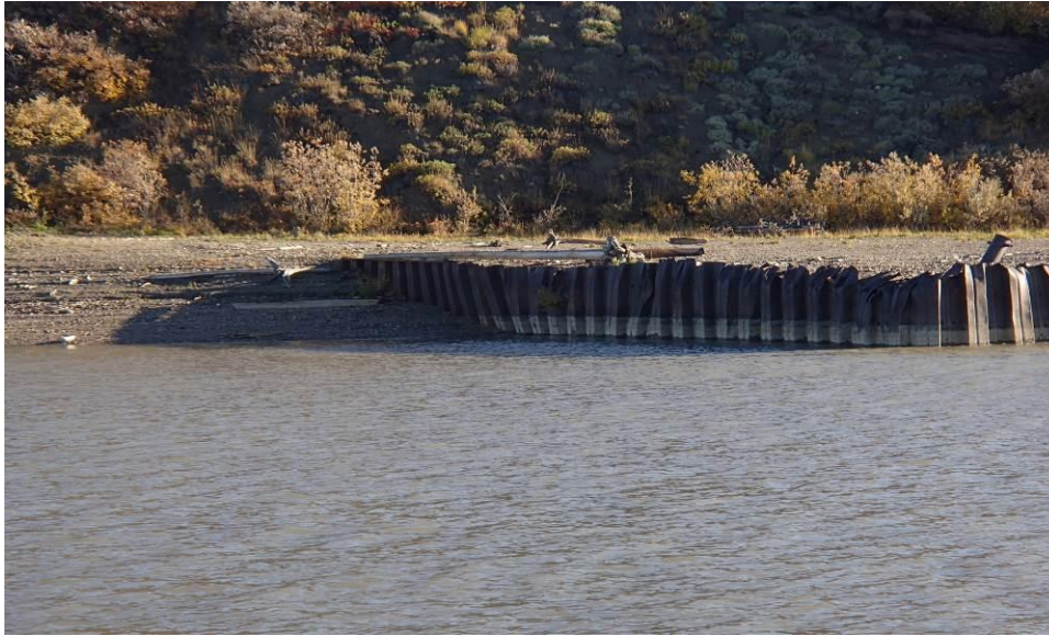
Photo 1: General view of the west wall.
