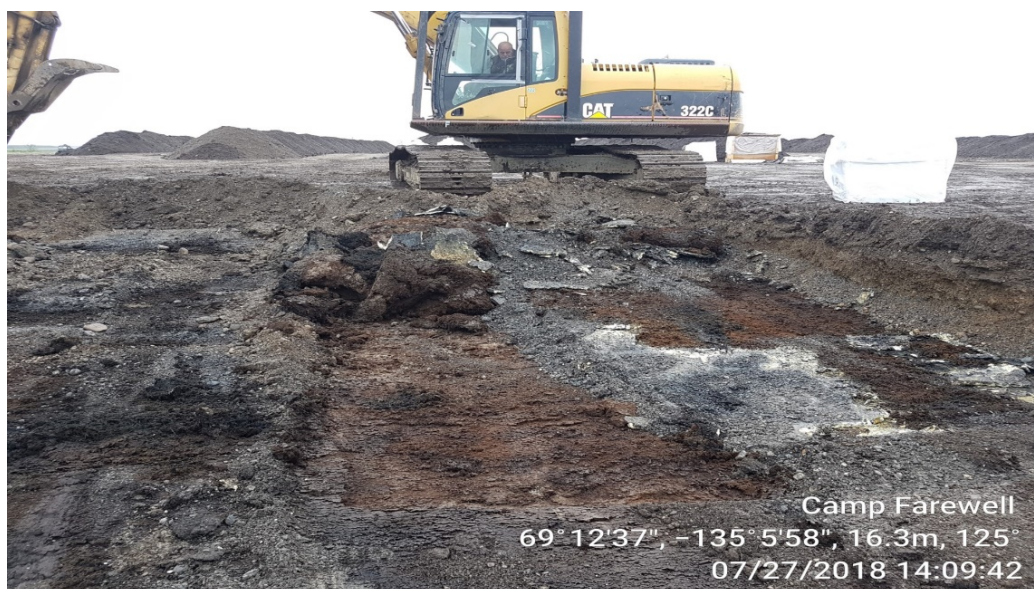
Photo 2 Excavating impacted fill and polyurethane foam overlying native peat (July 27, 2018).
