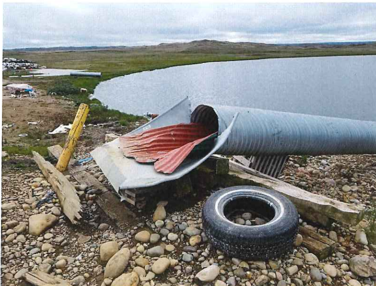
Figure 5 Unsafe Sewage Truck Chute, Poor Foundation
