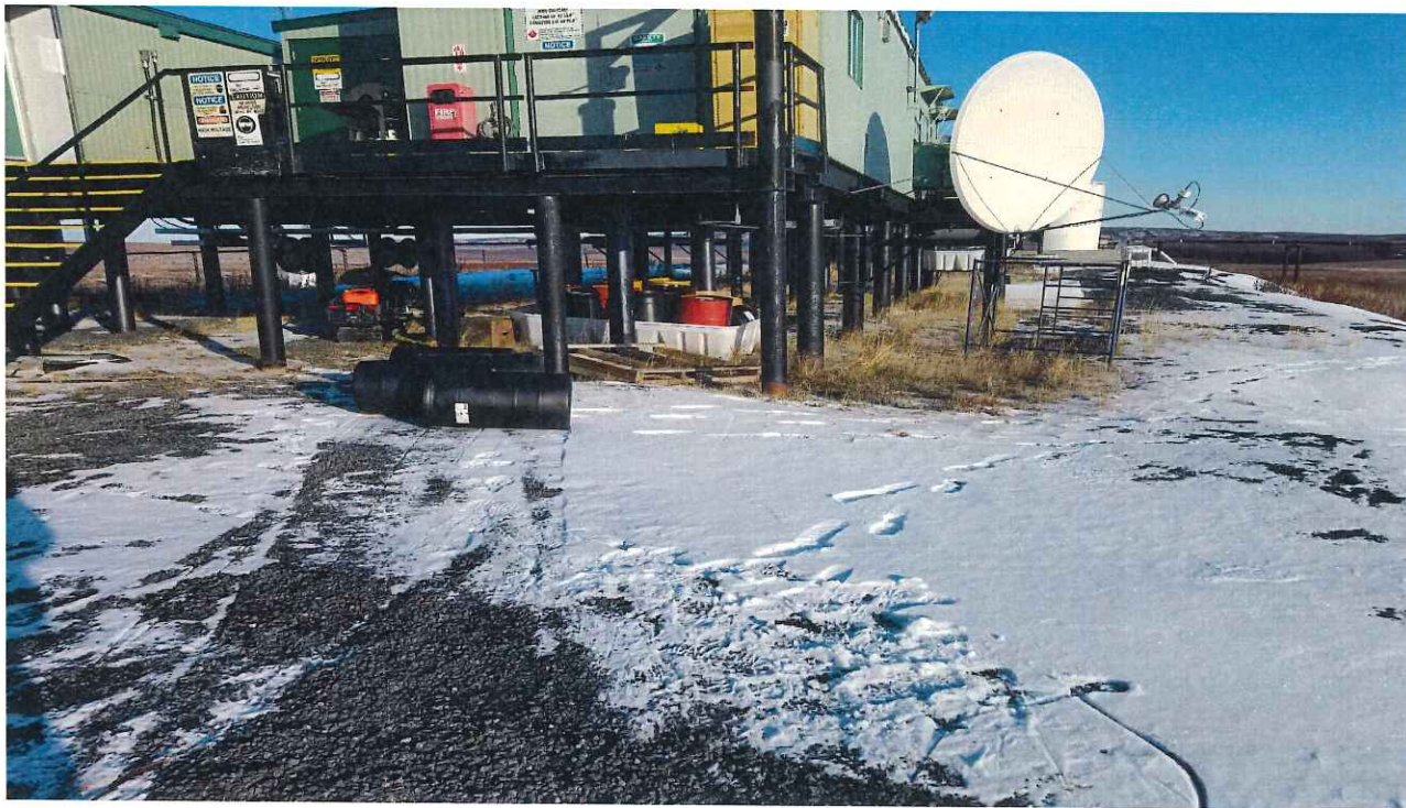
Figure 2 Picture facing east. No concerns with area
