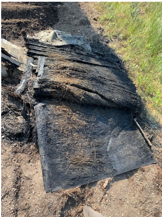
Photo 6 Waste materials (straw and fibreglass) encountered in Excavation #3.
