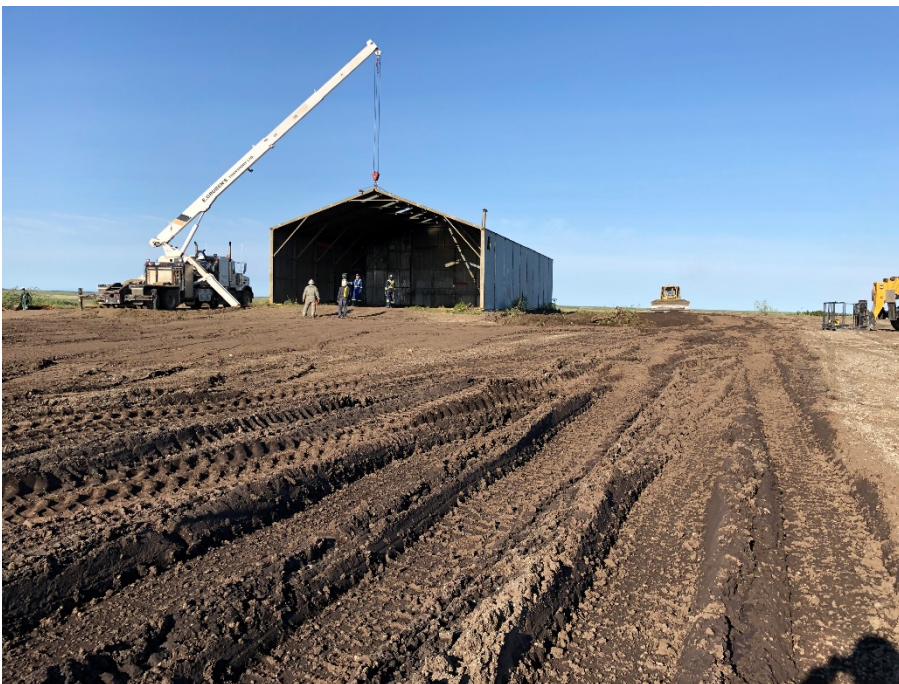
Photo 2 Dismantling of Shed #1 with Picker Truck.
