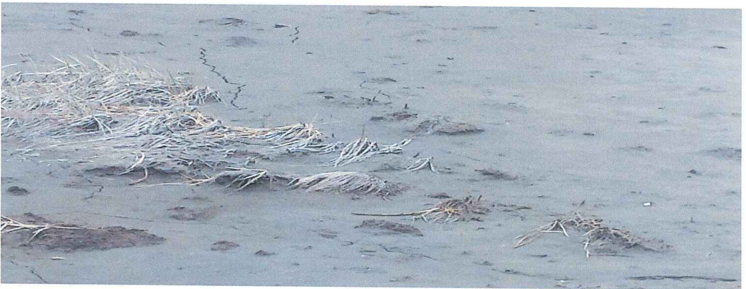
Figure 2 Cracking on new sump cap, July 21, 2020
