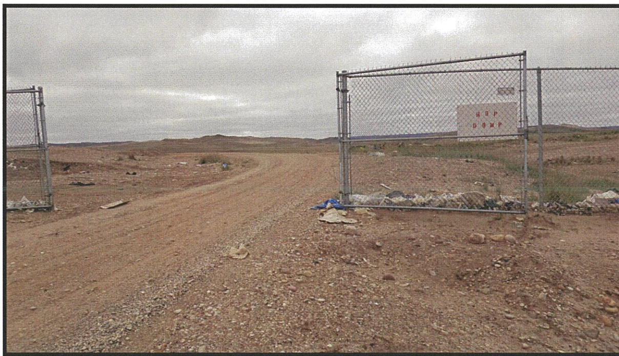
Photo 6: Access Road to Solid Waste Disposal Facility, Only Signage at the Facilities
