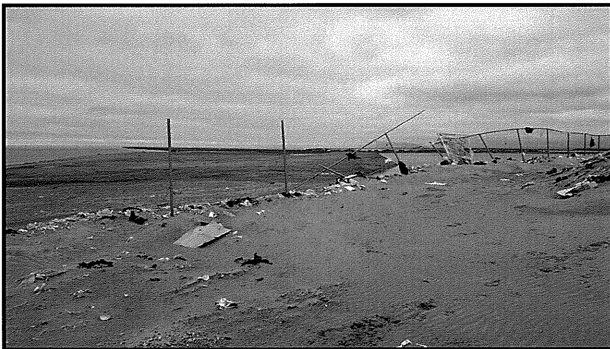
Photo 7: Downed Fence East of the Access Road, Looking North
