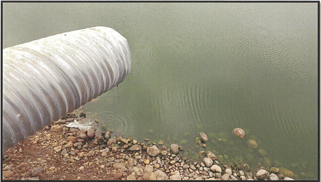
Photo 1: Sewage Lagoon Discharge Chute Outlet
