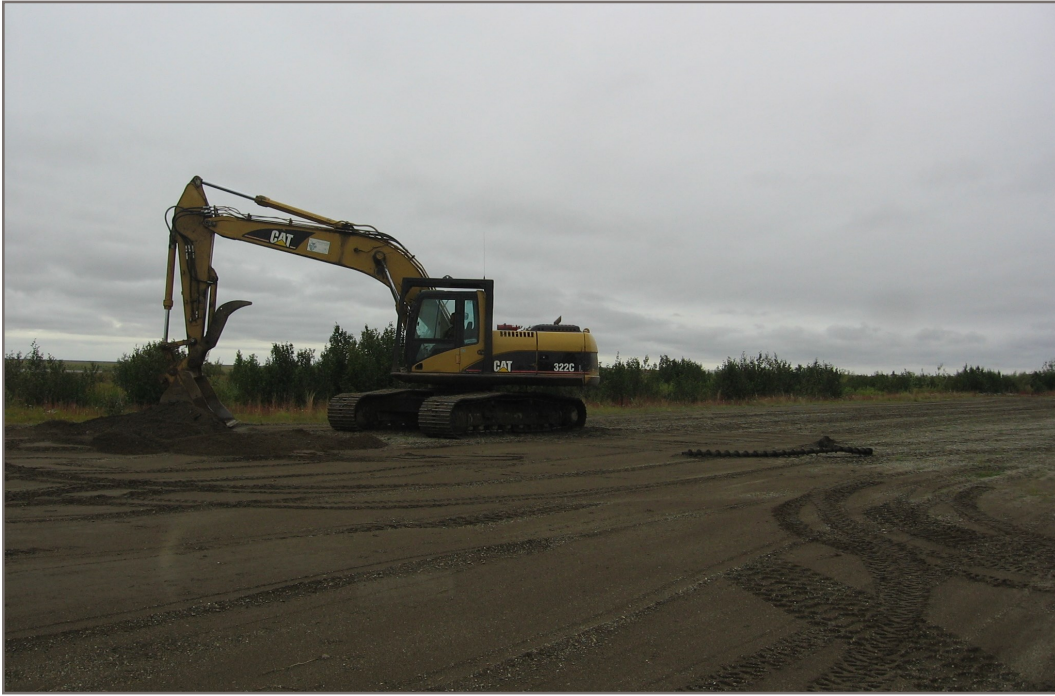
Photo 17: Geophysical anomaly Rwy7, post-excavation.
