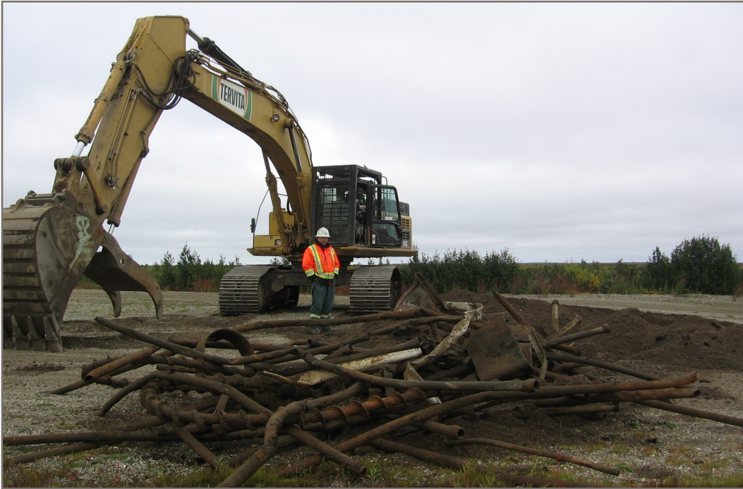
Photo 15: Geophysical anomaly Rwy1, post-excavation.
