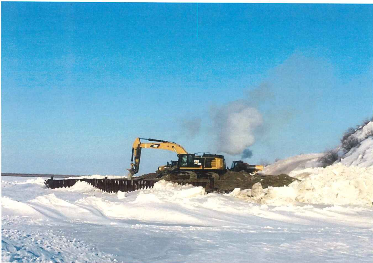
Dock removal work
