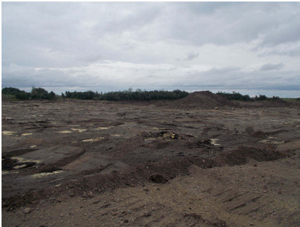
Photograph 2: View northwest of Zone 2 excavation (August 29, 2016).
