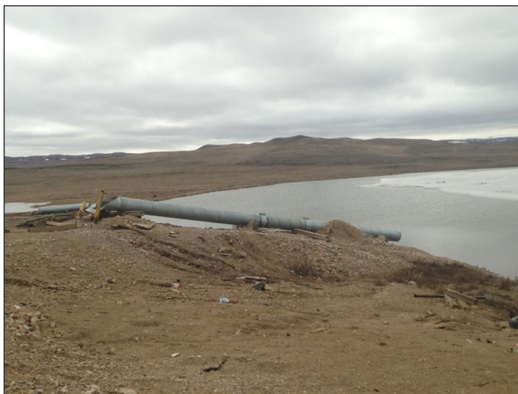
Figure 2: Paulatuk Discharge Chute (2015)
