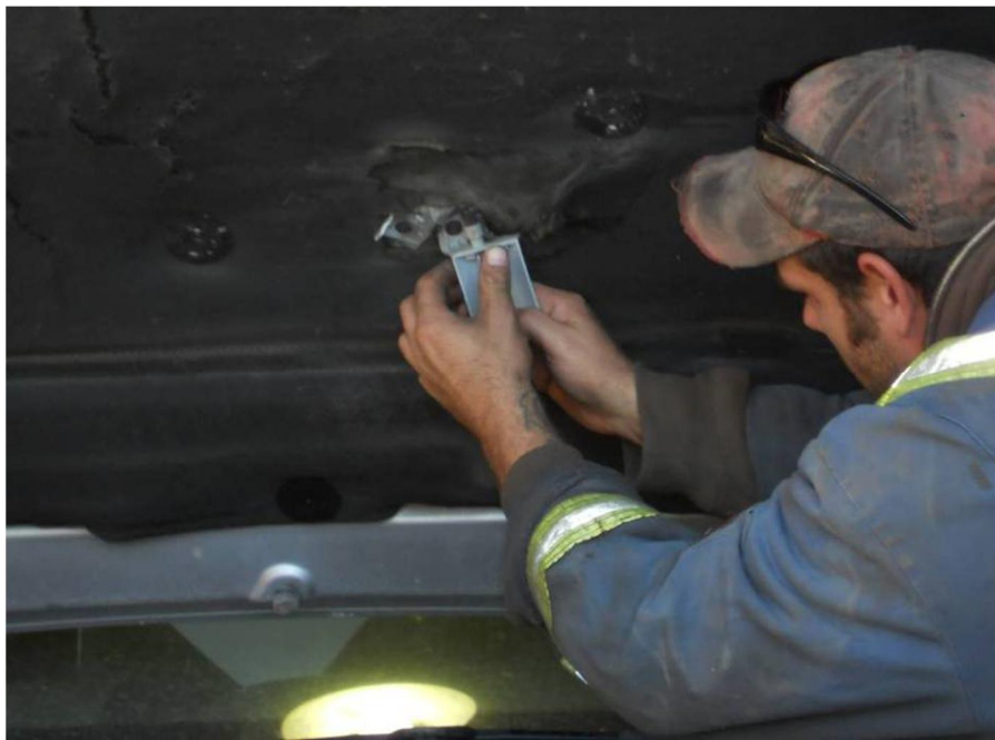
Figure 16: Example of Removing Light Assembly Containing a Mercury Switch
