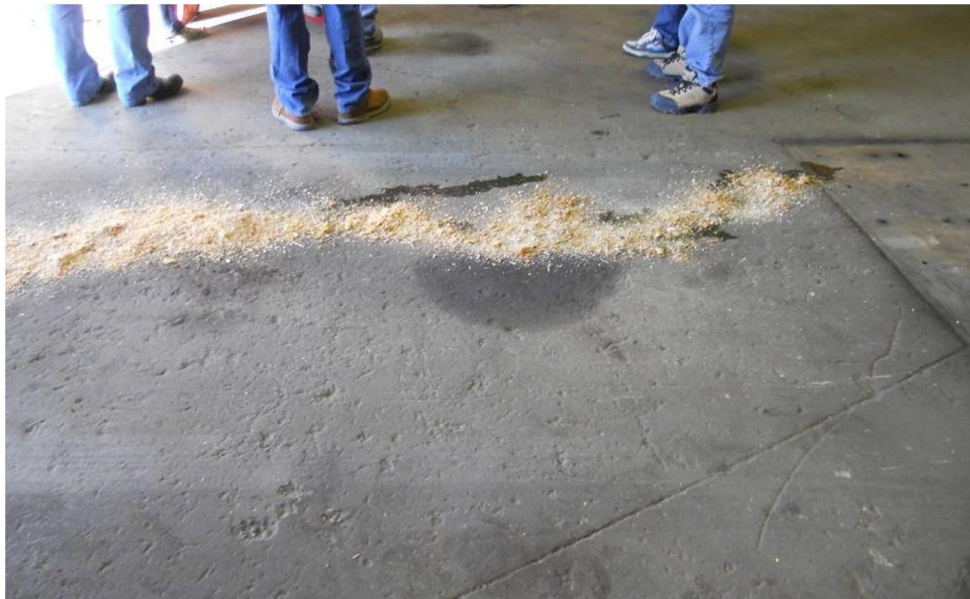
Figure 4: Absorbent Material Placed over Spilled Vehicle Fluids
