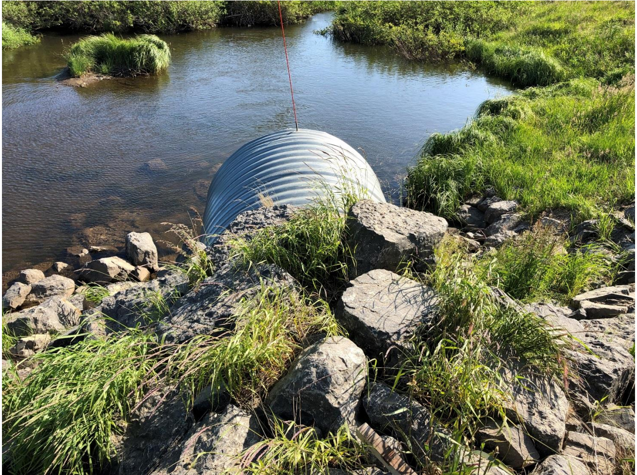
Figure 2-3 Gunghi Creek Crossing at km 131.2 ITH (No. 10) looking downstream
