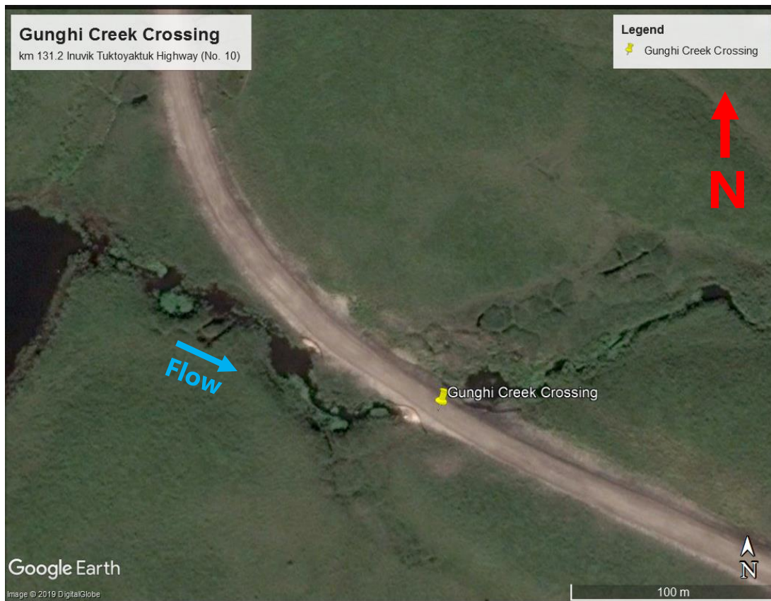
Figure 2-1 Gunghi Creek Crossing at km 131.2 ITH (No. 10)
