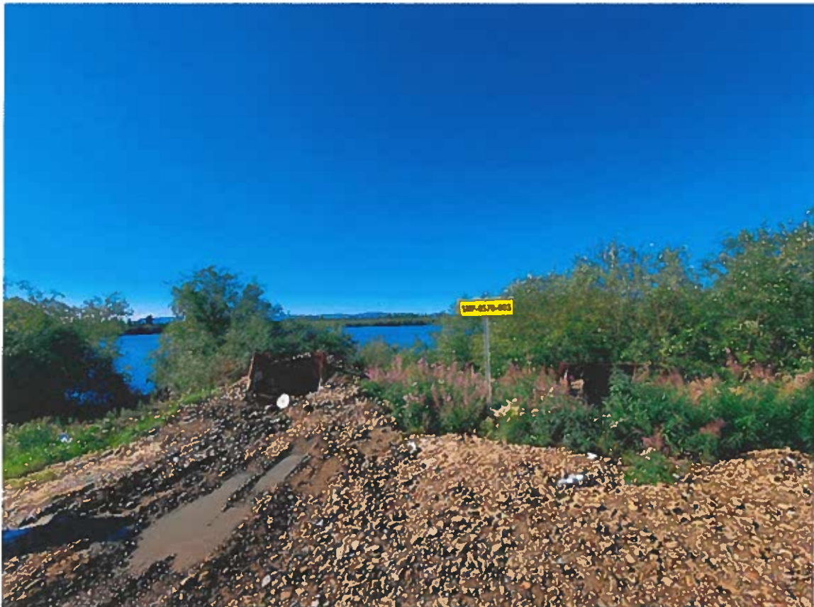
Figure 2 - Sewage Spill at the Sewage Waste Disposal Facility
