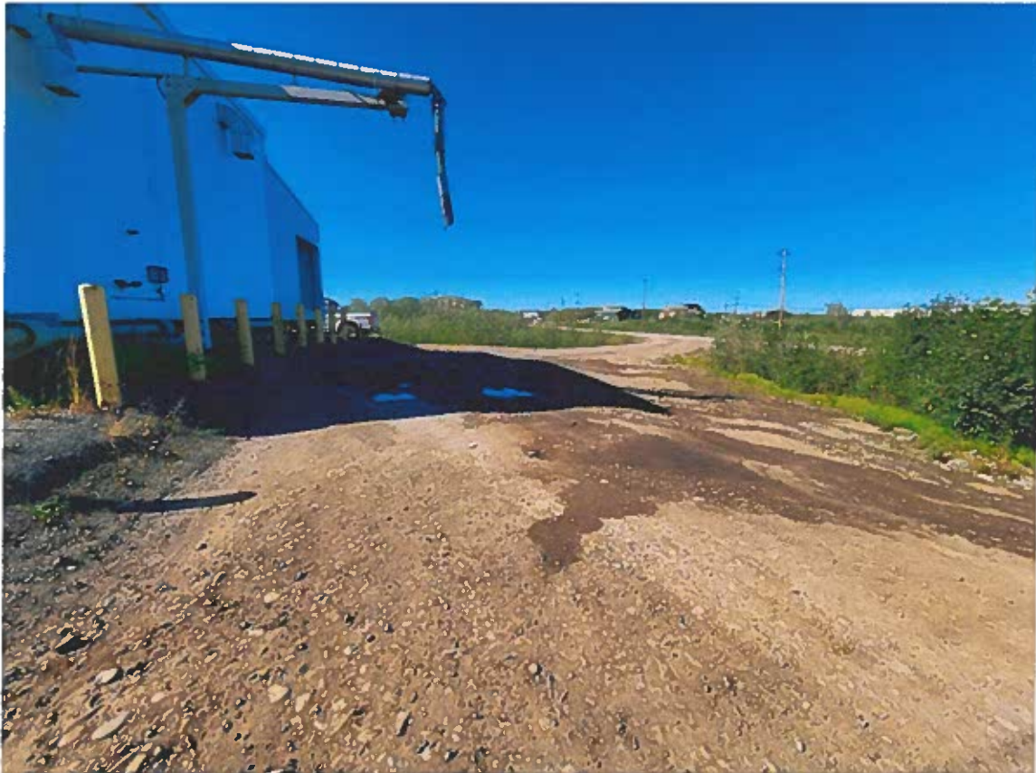
Figure 1 - Access Road to Water Treatment Plant
