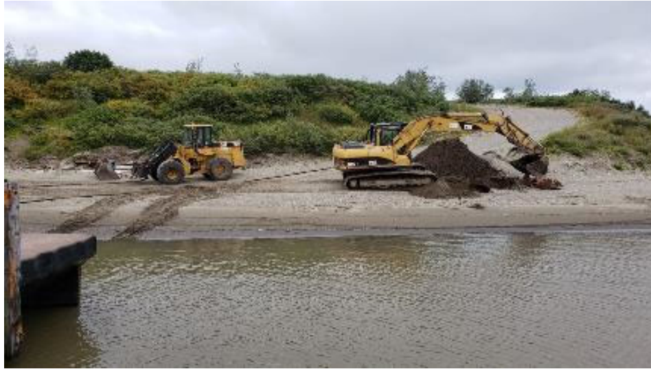
Photo 1 – Camp Farewell – Anchor installation (August 9, 2021).
