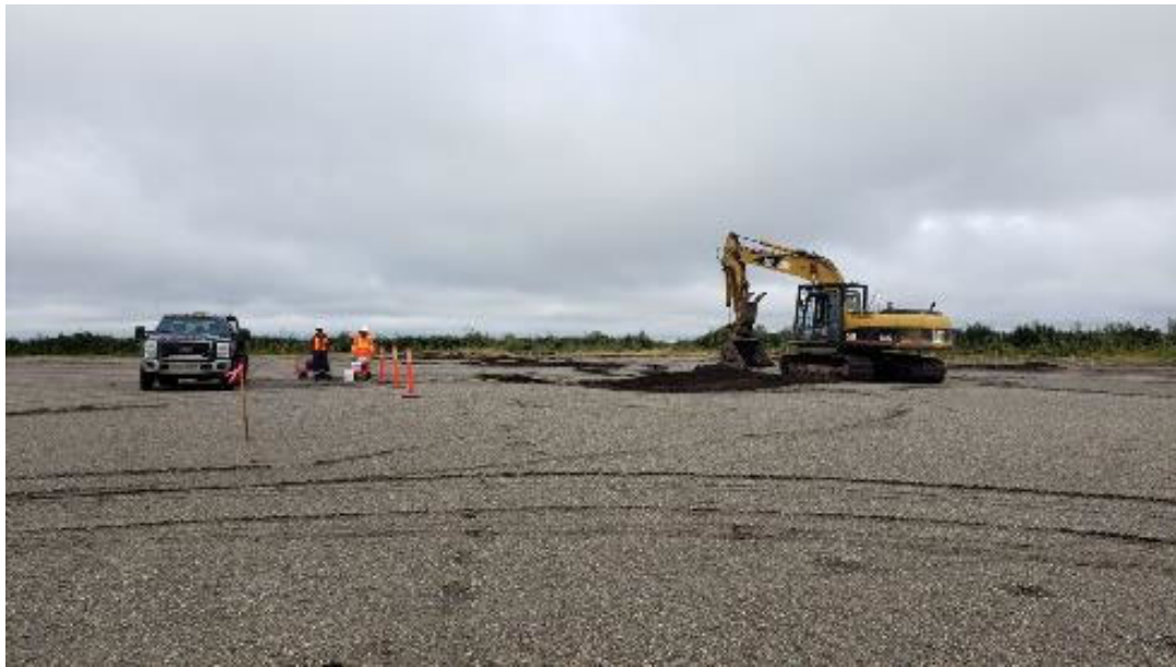
Photo 12 – Camp Farewell – Test pitting (August 16, 2021).
