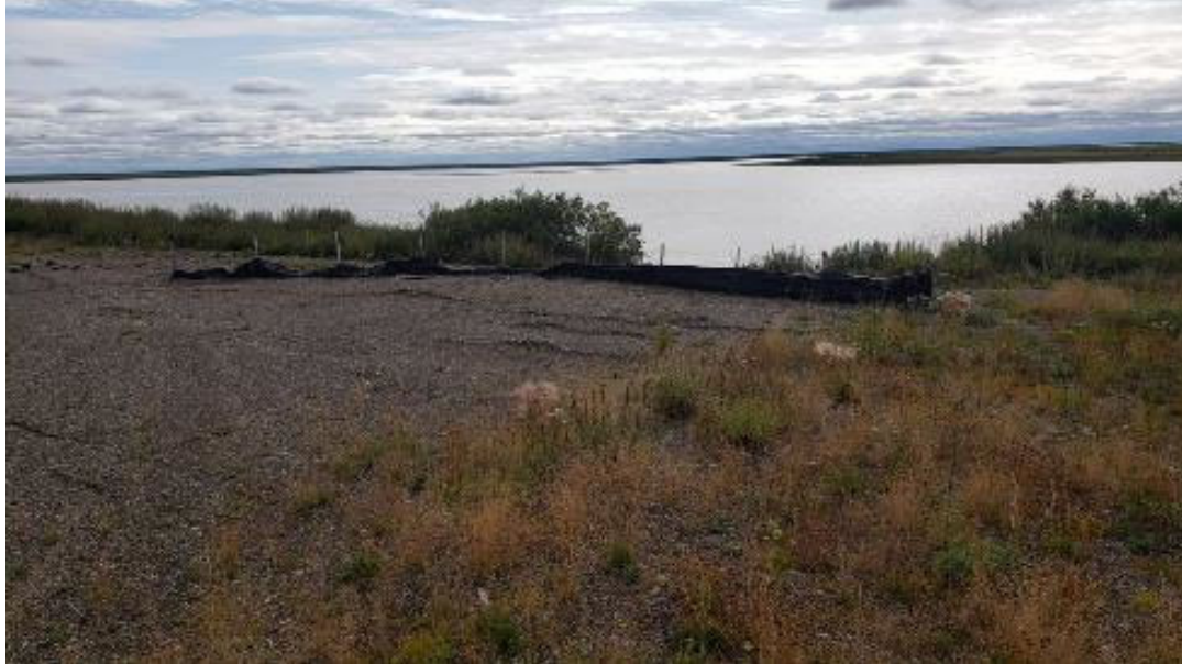
Photo 9 – Camp Farewell – Erosion control, facing south towards the Mackenzie river (August 13, 2021).
