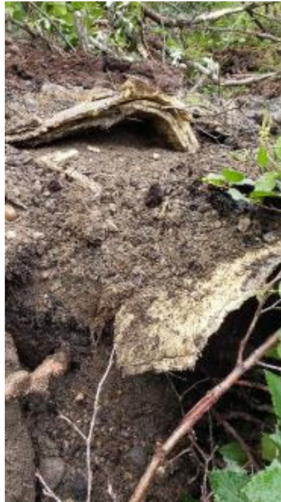
Photo 13 – Camp Farewell – Buried fiberglass material found in the north area of the Site (August 19, 2021).
