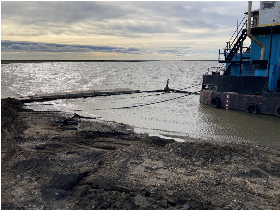
Photo 10 – View of the floating dock for the emergency boat on the east side of the barge camp, facing southeast (August 9, 2022).
