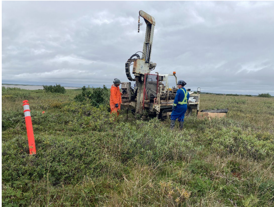
Photo 5 – Drilling at BH22-42, facing northwest (August 6, 2022).
