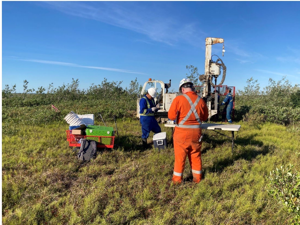
Photo 12 – Labelling soil samples at BH22-15, facing west (August 12, 2022).
