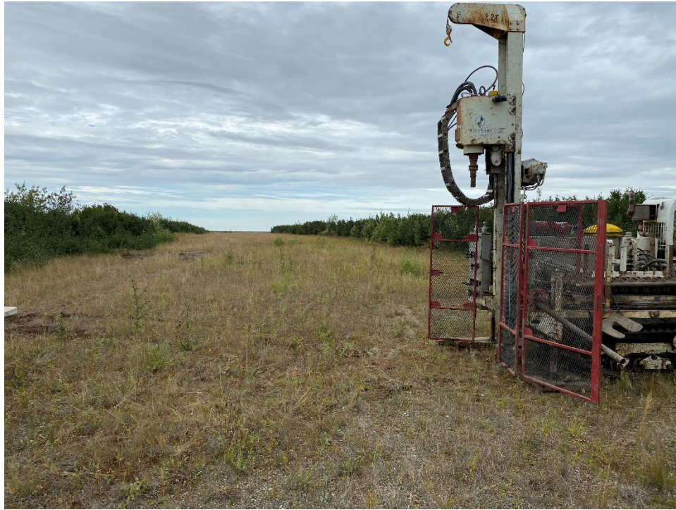
Photo 15 – Drill rig at BH22-65 on the former airstrip, facing northwest (August 24, 2022).
