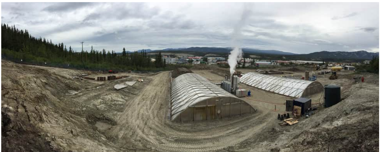
Photo 2: An operating ETC system with a quench tower connected to the process exhaust.
