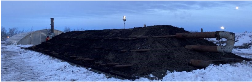
Photograph 1. ETC cell construction (West Channel Site).
