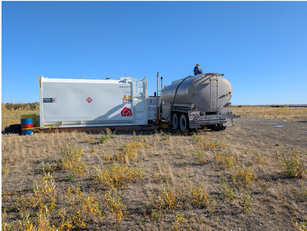
Photo 7 – Emptying fuel tank prior to demobilization, facing east (3 September 2025)
